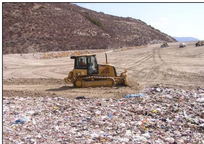
Figure 22 - Bulldozer placing cover soil on exposed waste.
