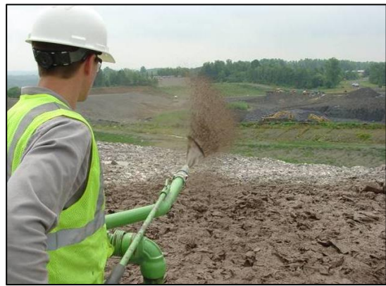
Figure 27 - Spray-on cement-based ADC.
