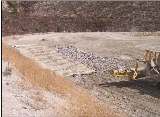
Figure 23 - Bulldozer placing ADC (tarp) on exposed waste.
