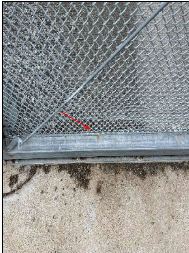
Photo 10. Gap in the wire mesh at the western gate west of the ACC, first observed on April 15, 2024.
