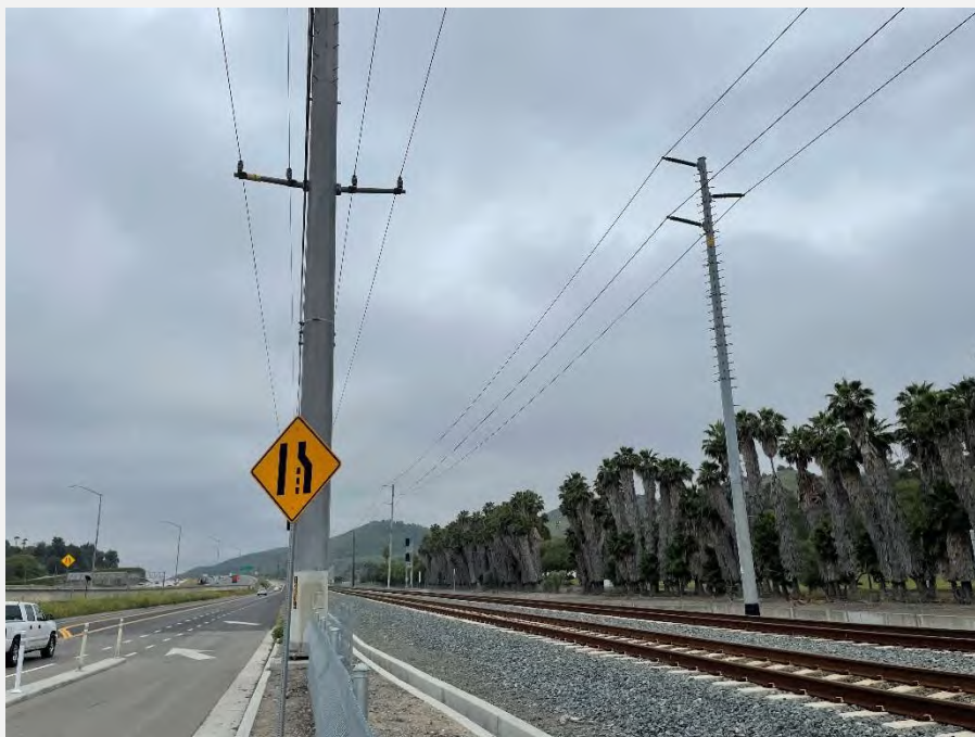
Photo 3. Transmission Line, steel tubular poles, looking south.
