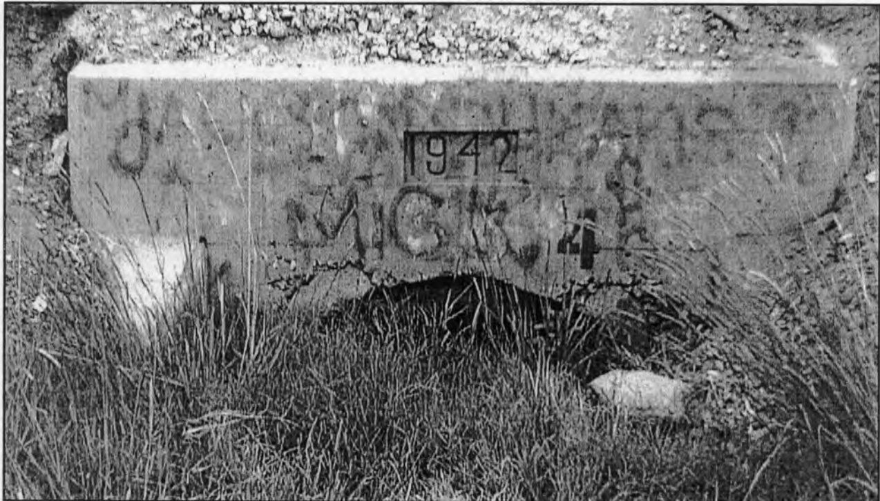
Old concrete culvert across the railroad bed
