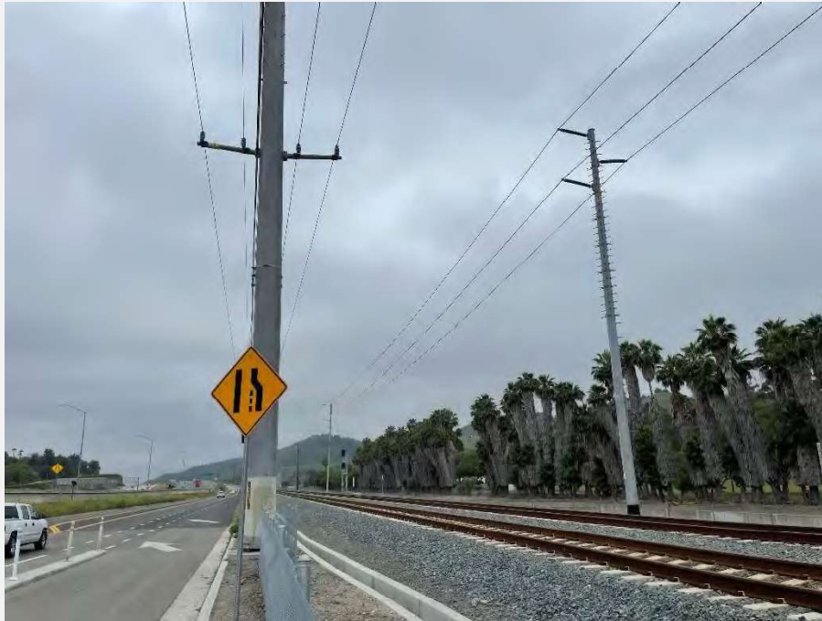
Photo 3. Transmission Line, steel tubular poles, looking south.
