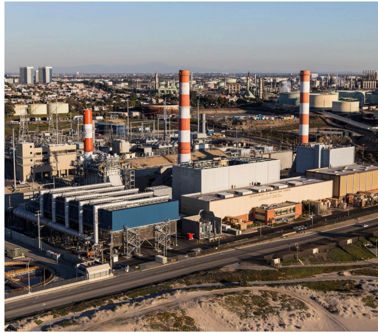
Scattergood Generating Station, Los Angeles
