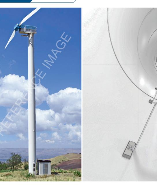
Some wind-turbine manufacturers have developed magnetic mounting systems that securely attach ladders and other equipment to the steel tower walls. (Courtesy: Amazing Magnets)
