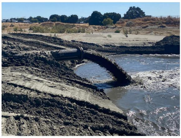
**Photo 3.** Pipe pumping dredged sand material from the San Juaquin River into Management Area 2 of the Stamm Unit.
