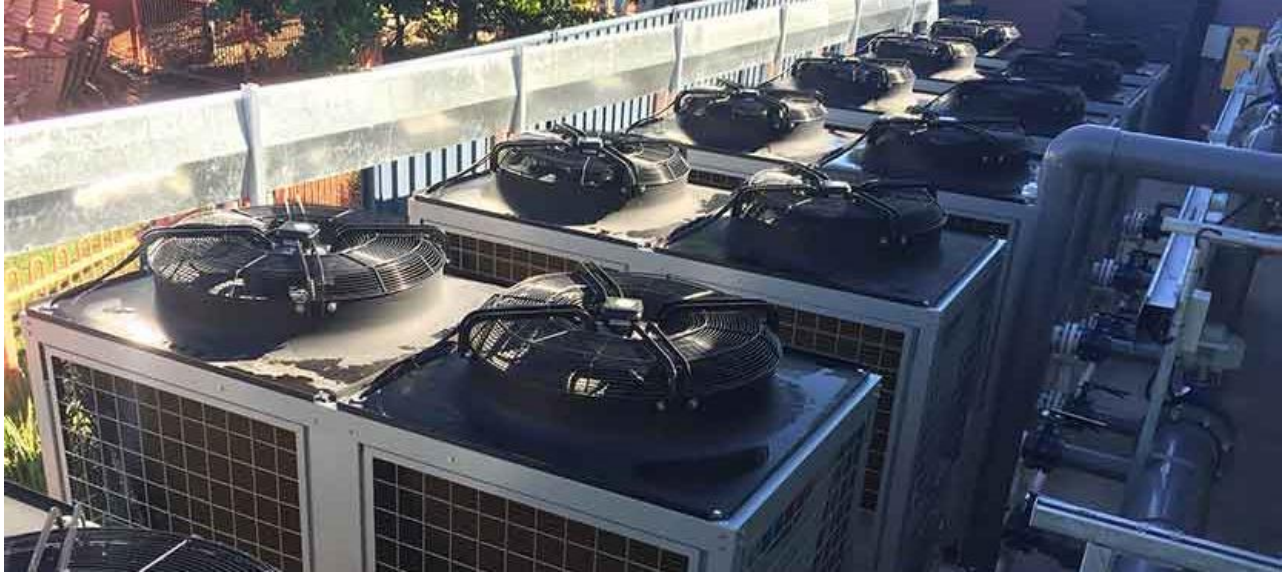
Figure 5: Bank of HPPH for Large Aquatic Center
