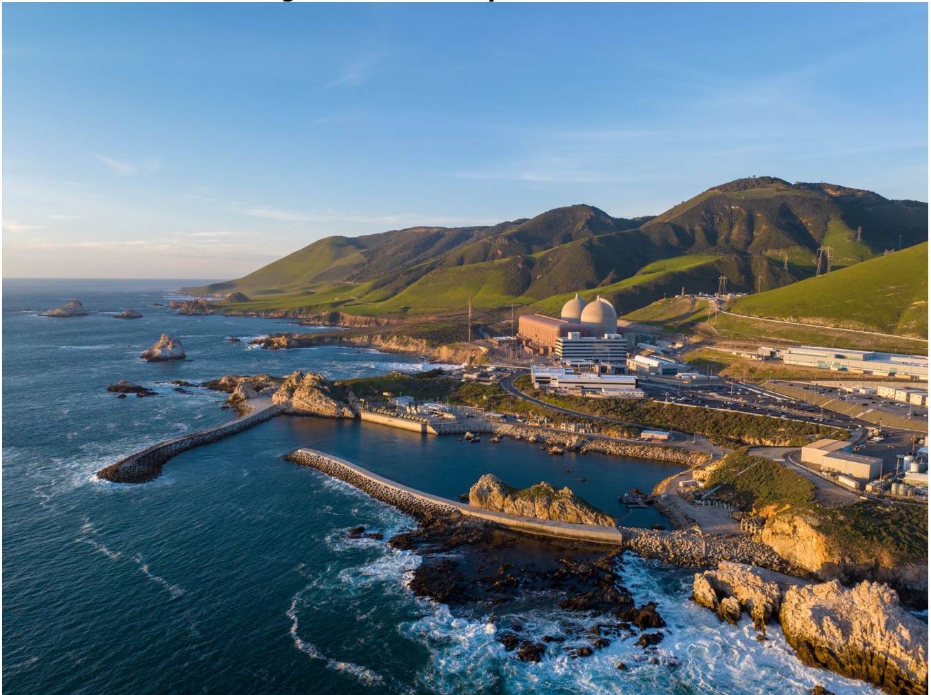
Figure 1: Diablo Canyon Power Plant
