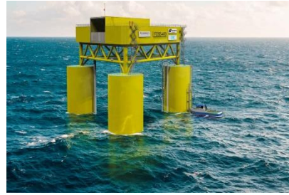
Semco Maritime, ISC Consulting Engineers, and Technip Energies' three-column stabilized substructure design, FOSS-400 37
