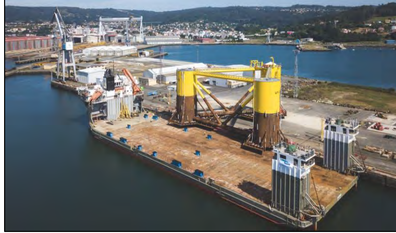
2) Loadout onto semi sub
