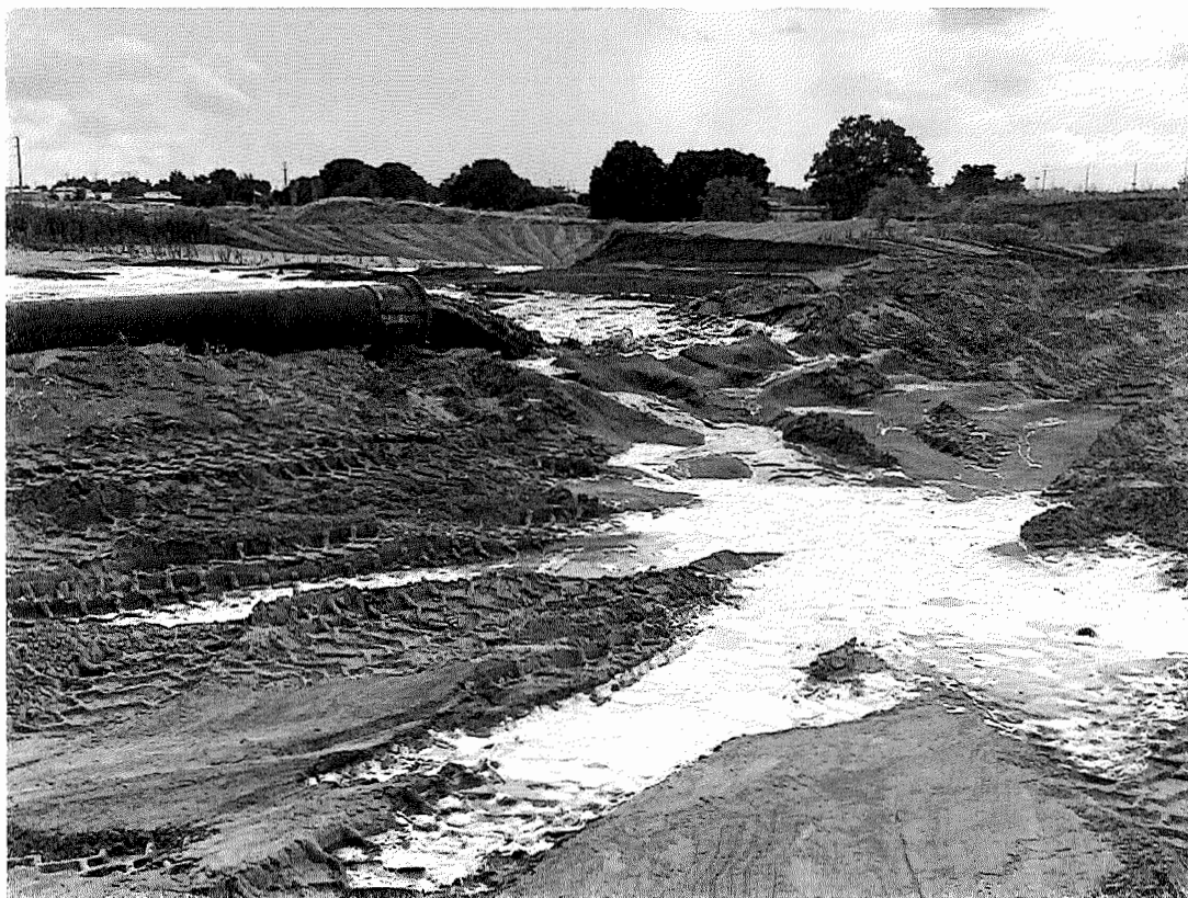
Photo 3. Pipe pumping dredged sand material from the San Joaquin River into Management Area 2 of the Stamm Unit.
