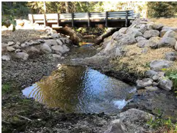
Photo 26. Cedar Creek, a perennial stream (data points 42-44). Adjacent riparian wetlands are recovering from a recent bridge installation. Orientation: southwest.
