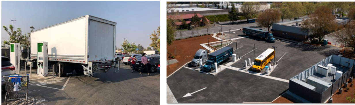
Figure 2. Example of medium-duty vehicle attempting to utilize existing EV infrastructure catering only to light-duty passenger vehicles (left), resulting in traffic disruption and operator frustration. Portland's Electric Island (right) shows successful implementation of dual purpose pull-through charging infrastructure able to support all vehicle classes.
