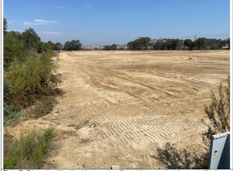
**Photo #7:** This is a view of the old tank farm area where fill materials was stored and then used to fill in the tunnels and below-grade areas. It was estimated that over 100,000 cubic yards of fill was placed. This area is clean and well-graded.
