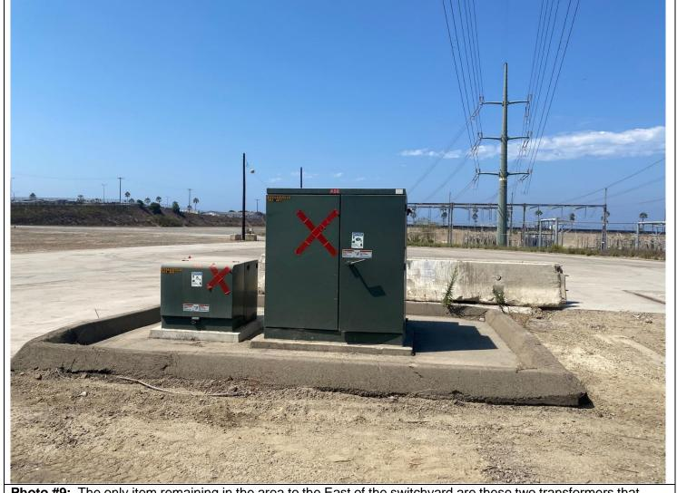
**Photo #9:** The only item remaining in the area to the East of the switchyard are these two transformers that belong to SDG&E. They have been drained and decommissioned and SDG&E has been notified that they can be removed at any time.
