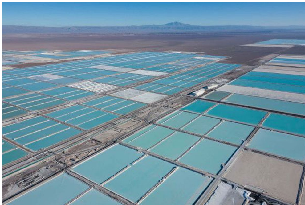
Figure 6: Lithium Evaporation Ponds in San Pedro de Atacama, Chile
