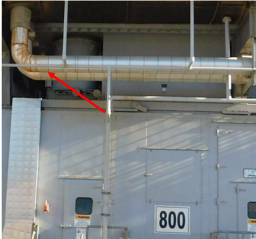
Figure 5. Brown fluid stain (indicative of a leak) observed at Unit 800, underneath air intake.
