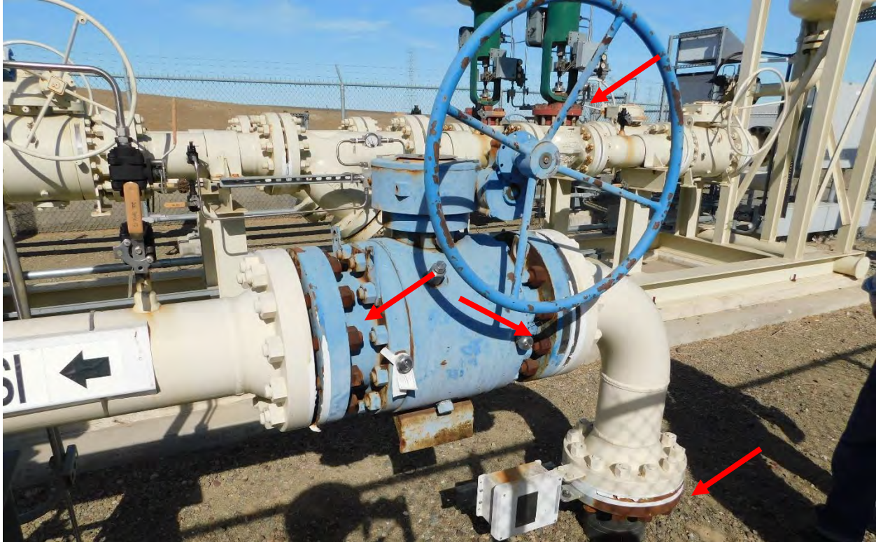
Figure 2. Fuel Gas Yard pipe flanges and fasteners show signs of atmospheric corrosion.
