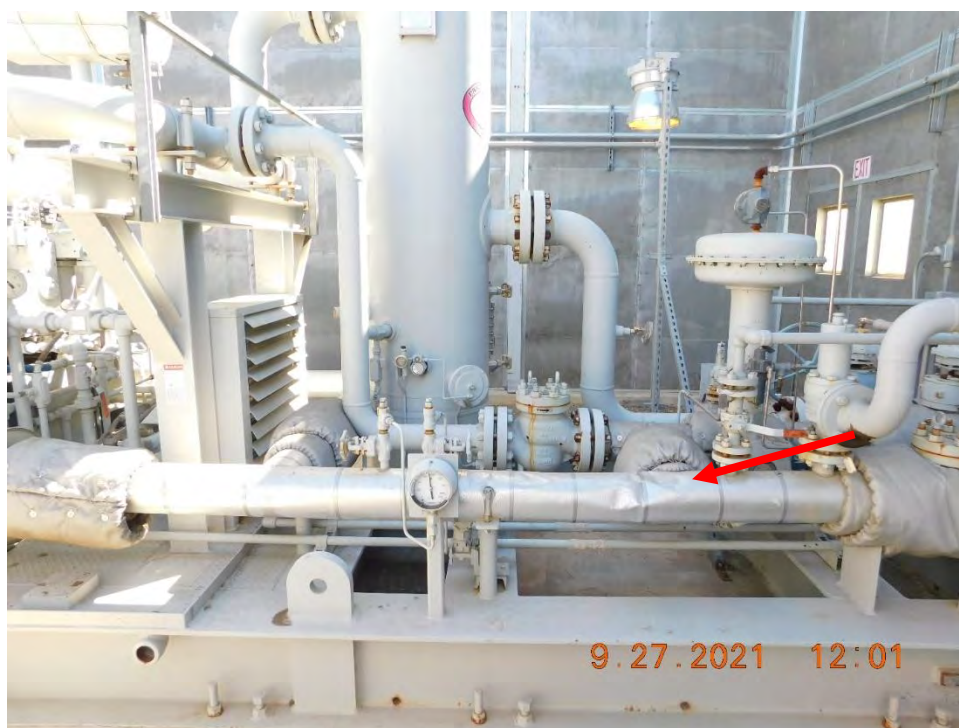
Figure 117. Damaged insulation and jacket in the Natural Gas Compressor building.
