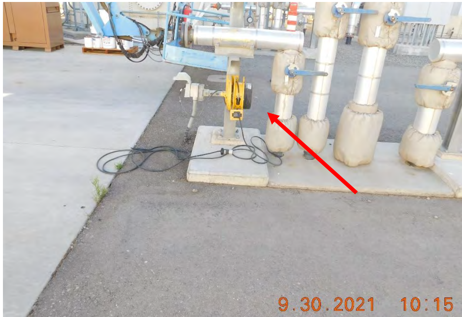
Figure 4. Broken cord reel was observed and later corrected.
