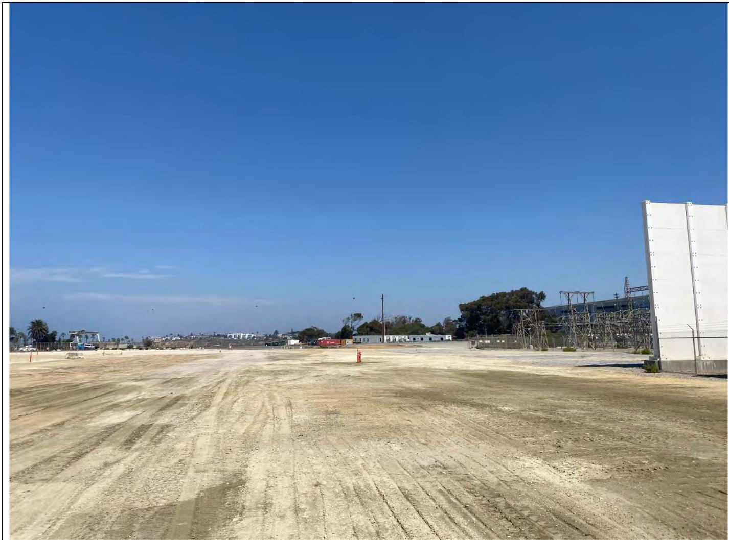
**Photo #13:** The area to the west of the switchyard is clean and graded to slope to the west.
