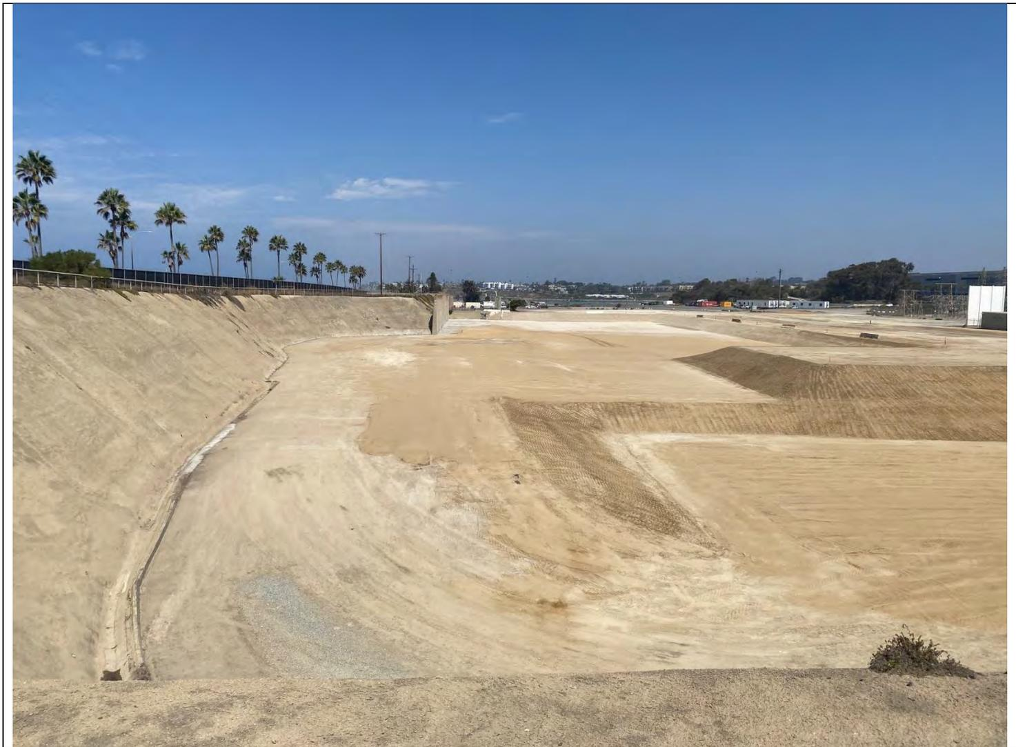
**Photo #11:** This photo was taken from the south road looking north. The entire area that housed Units 1-5 has been graded smooth and no foundations are showing. The site is sloped to drain to the south-east corner where existing sumps are provided.
