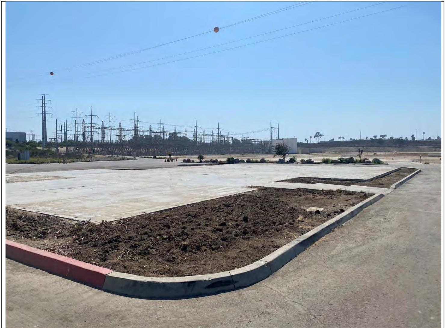
**Photo #1:** This image shows the slab-on-grade for the old administration/office building. The City Fire Department wanted the curbing and slab to remain for purposes of setting equipment and to provide parking.
