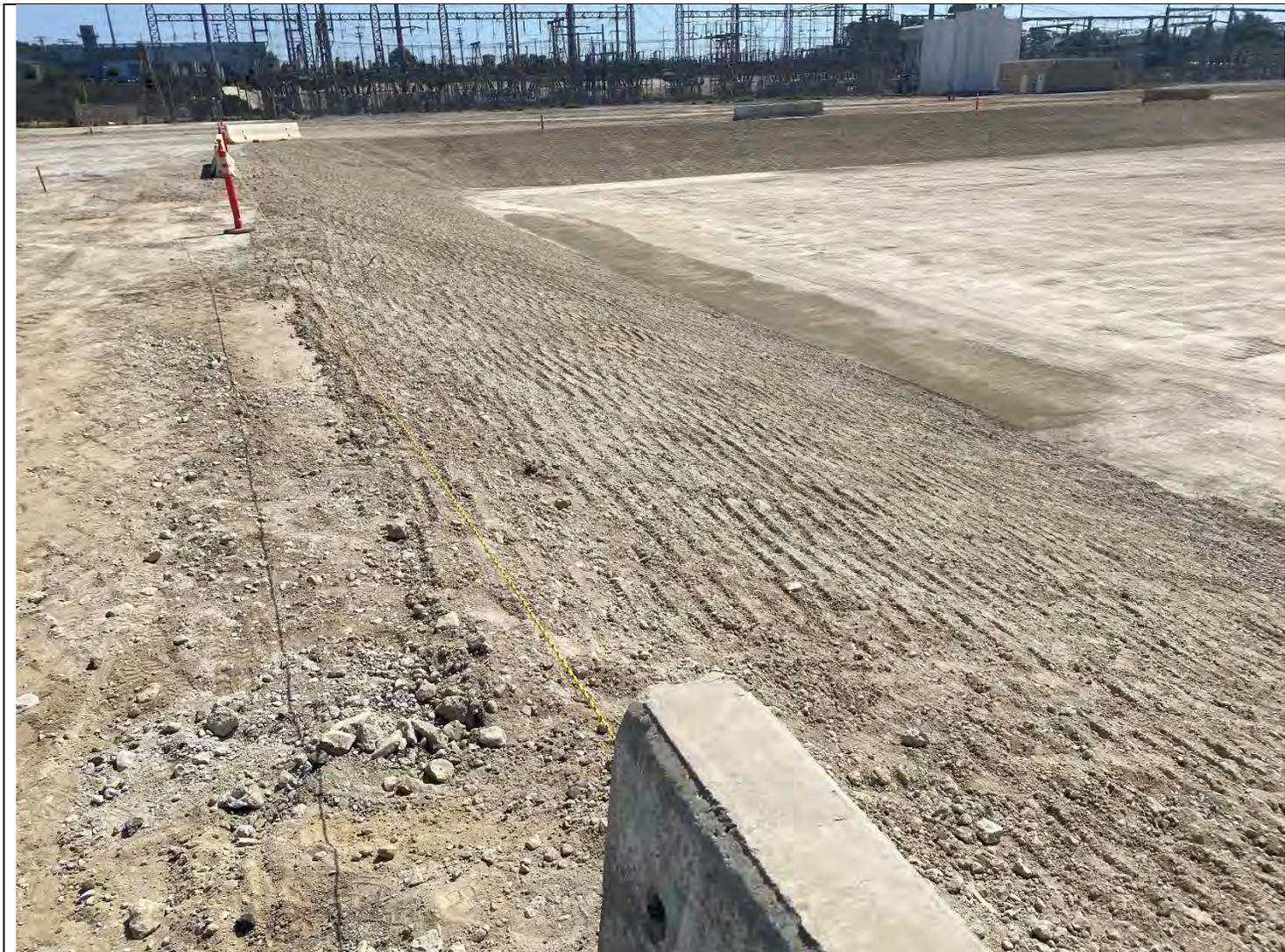
**Photo #6:** The sloped areas have K-barrier at the top with ropes to keep people or vehicles from traversing the slopes.
