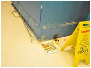
15. View of the floor drain for cooling equipment condensate within the 2710 Walsh Avenue building
