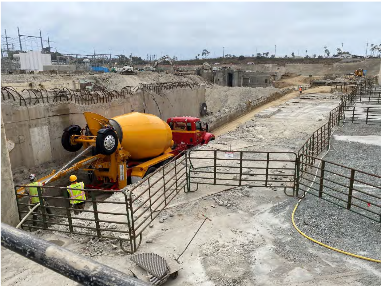
Photo #5: Here is a photo of a truck just completing the placement of some flowable fill.
