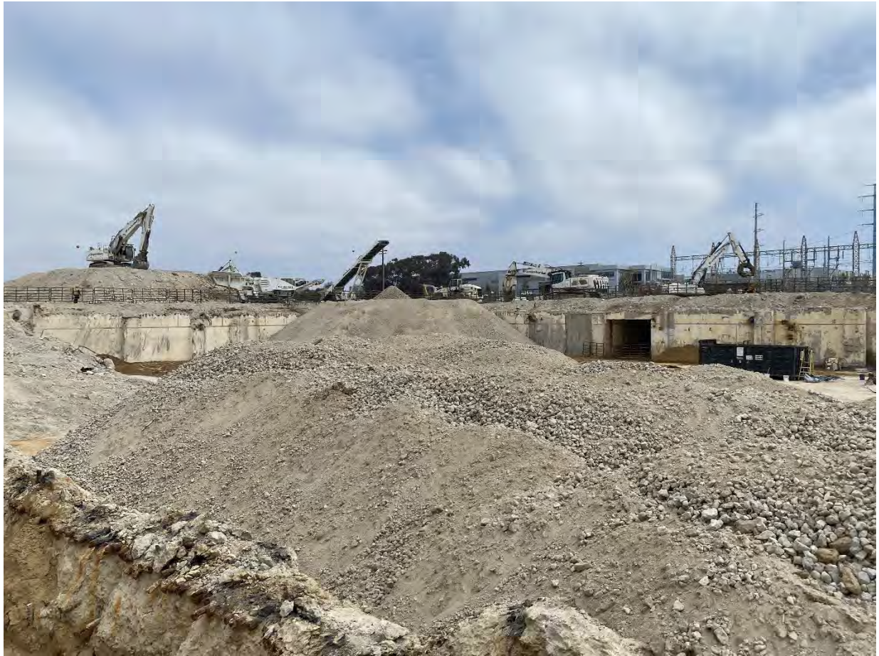
Photo #7: A geotechnical technician is onsite fulltime to verify the proper gradation of fill, ensure that the lift thickness has not been exceeded, and to ensure that 95% compaction is achieved.
