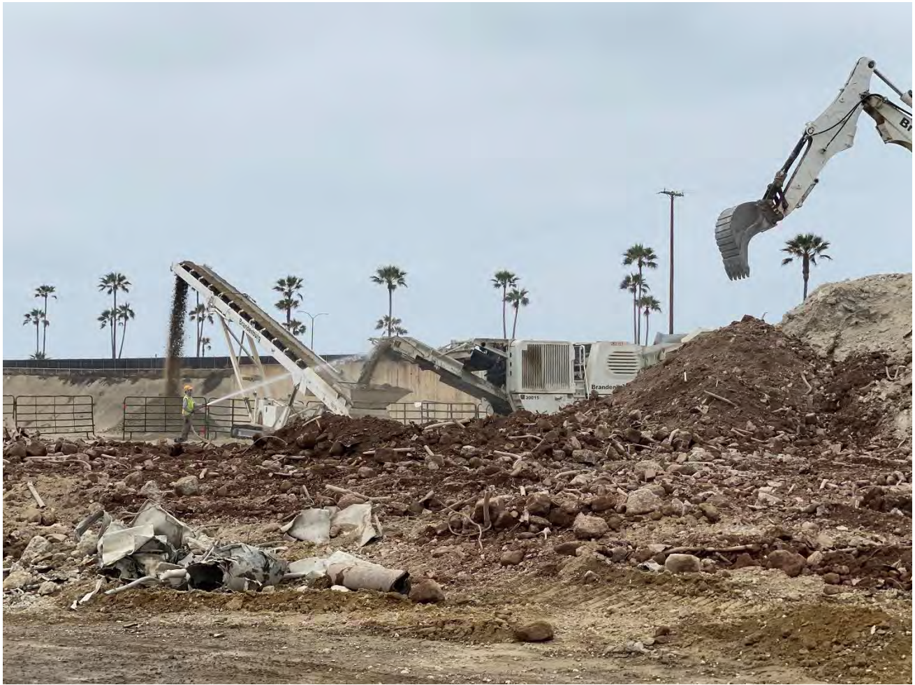
Photo #11: Fill from the site of the old tank farm is being used to bring the site up to grade. This photo shows the excavation of this fill area and trucks that take it to the demolition site.
