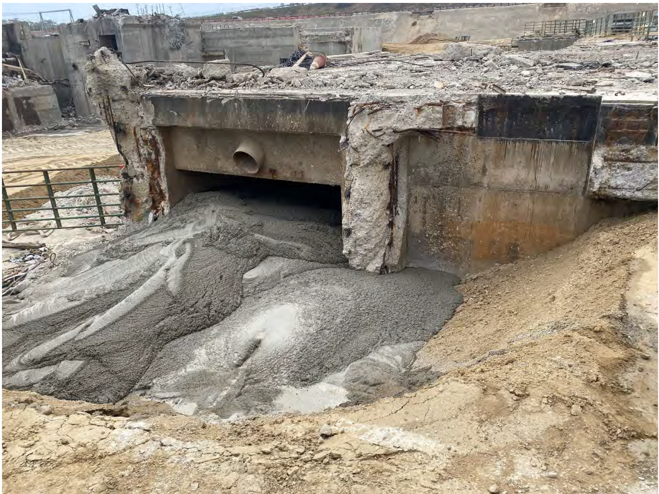
Photo #3: A large amount of flowable fill is being brought to the site to fill the tunnel areas as shown below.
