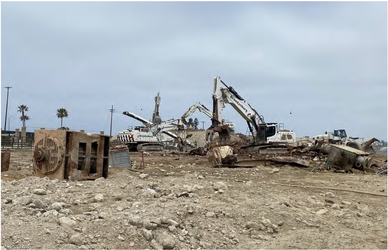
Photo #9: The concrete pile is sifted and as much metal as possible is removed prior to crushing.
