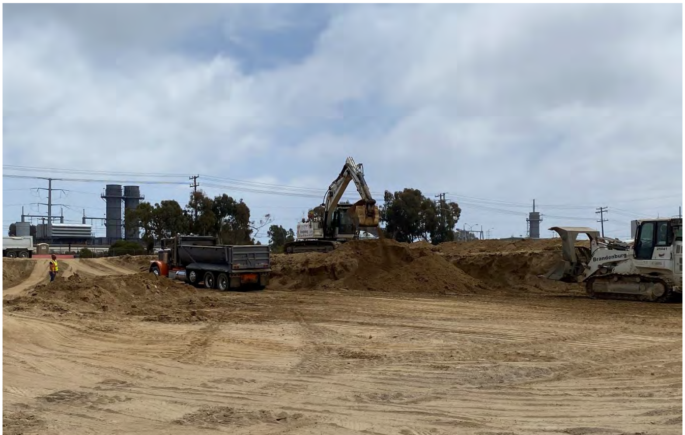
Photo #11: Fill from the site of the old tank farm is being used to bring the site up to grade. This photo shows the excavation of this fill area and trucks that take it to the demolition site.
