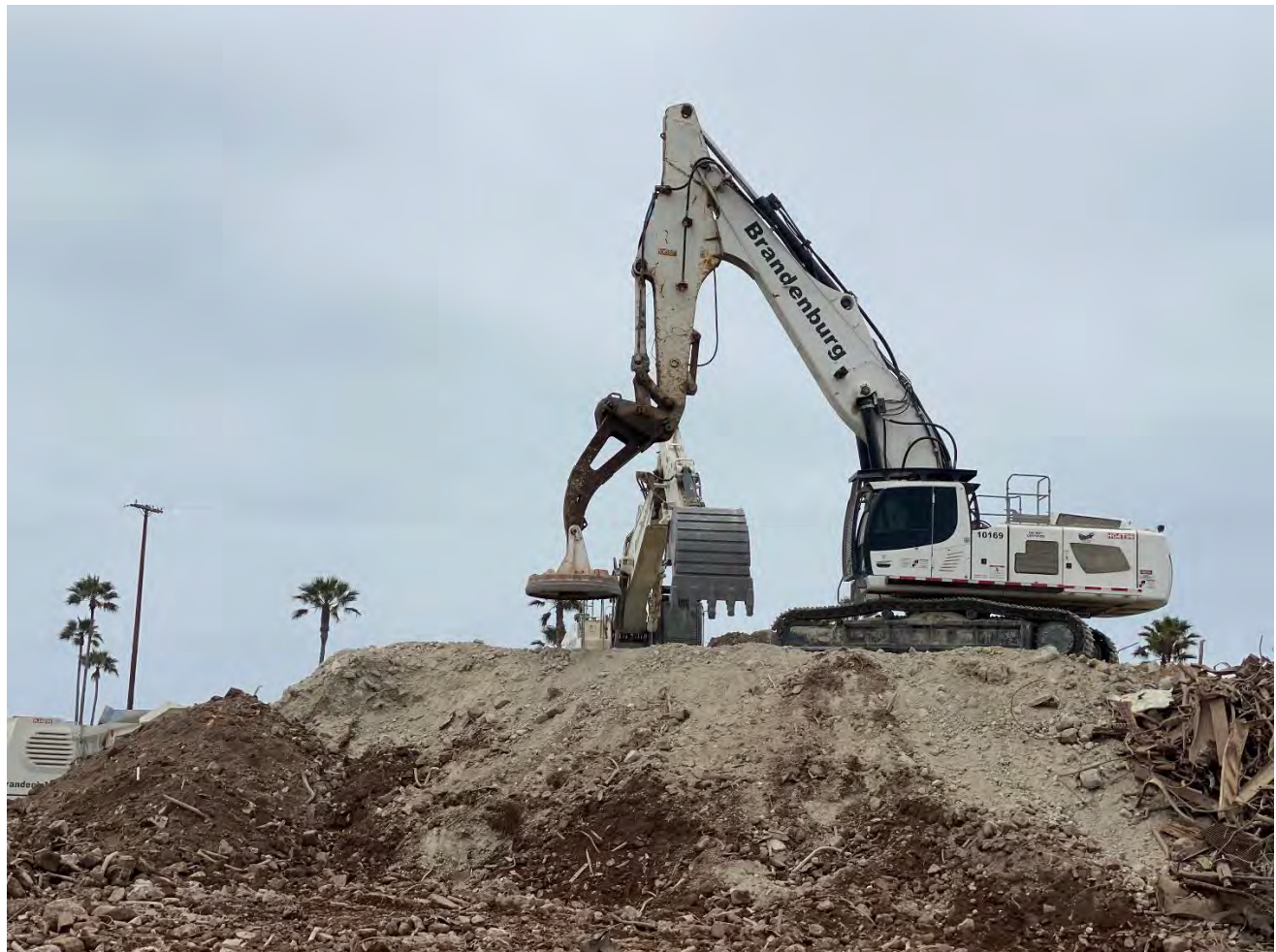
Photo #9: The concrete pile is sifted and as much metal as possible is removed prior to crushing.
