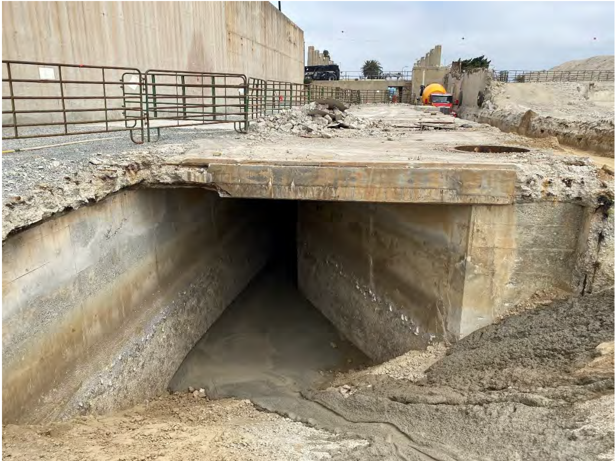
Photo #5: Here is a photo of a truck just completing the placement of some flowable fill.
