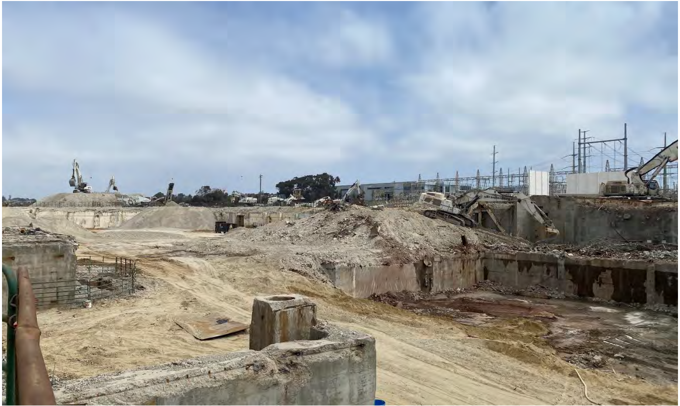
Photo #3: A large amount of flowable fill is being brought to the site to fill the tunnel areas as shown below.
