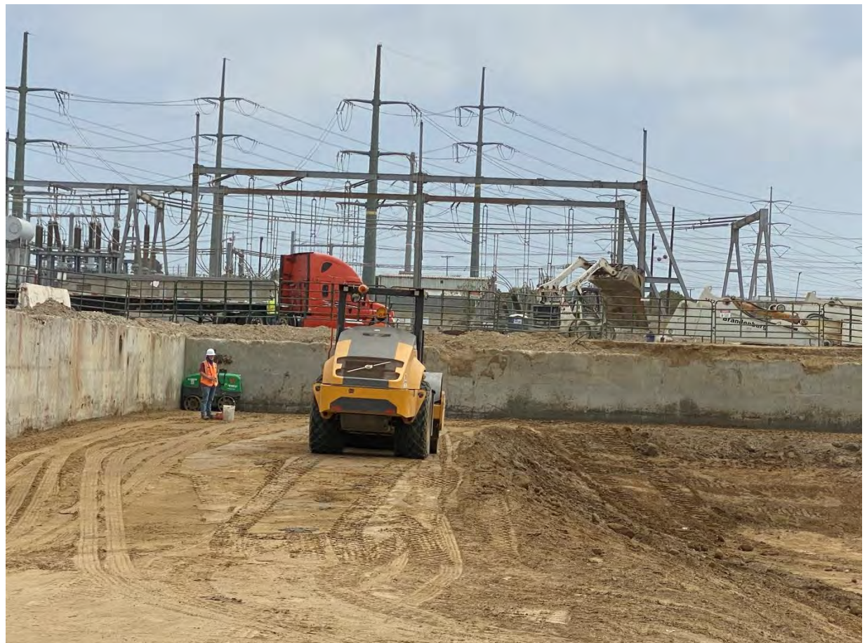
Photo #7: A geotechnical technician is onsite fulltime to verify the proper gradation of fill, ensure that the lift thickness has not been exceeded, and to ensure that 95% compaction is achieved.
