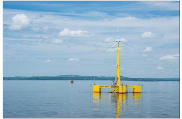
VolturnUS, 1:8 scale of a 6 MW wind turbine near Maine. VolturnUS was built at U Maine. It is the first grid connected offshore wind turbine in the US. (https://composites.umaine.edu/research/volturnus/)
