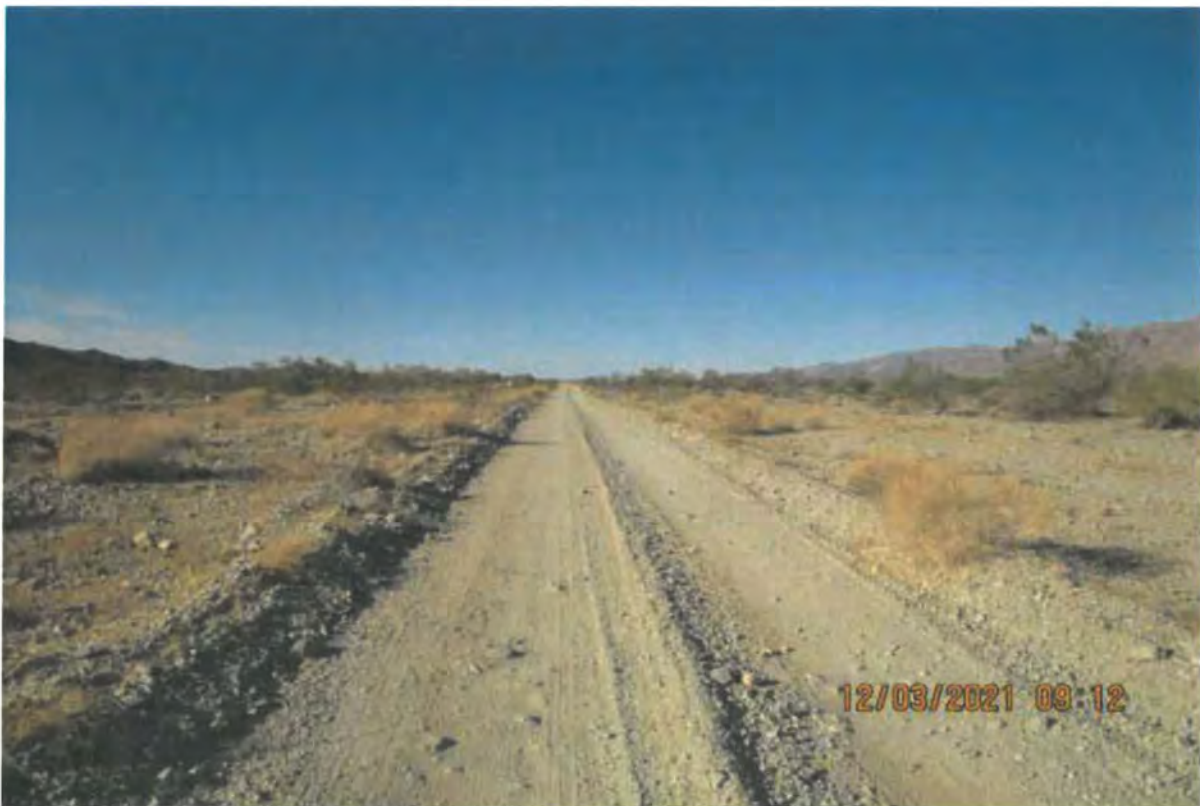
10. Looking southwesterly along the high-pressure natural gas pipeline that is adjacent (south) of the southeast corner of the Property (641,302mE, 3,729,859mN).
