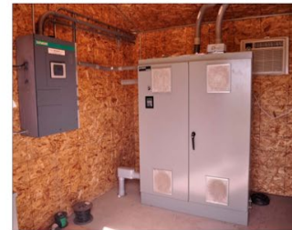
200 HP MOTOR STARTING VFD & 100 HP REGENERATION VFD WITH LOCAL CONTROL PANEL.
