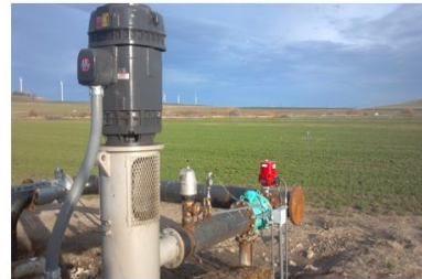
200 HP MOTOR WITH VERTICAL LINE SHAFT PUMP – 8" PIPE, AQUIFER LEVEL 520 FEET BELOW LAND SURFACE.
