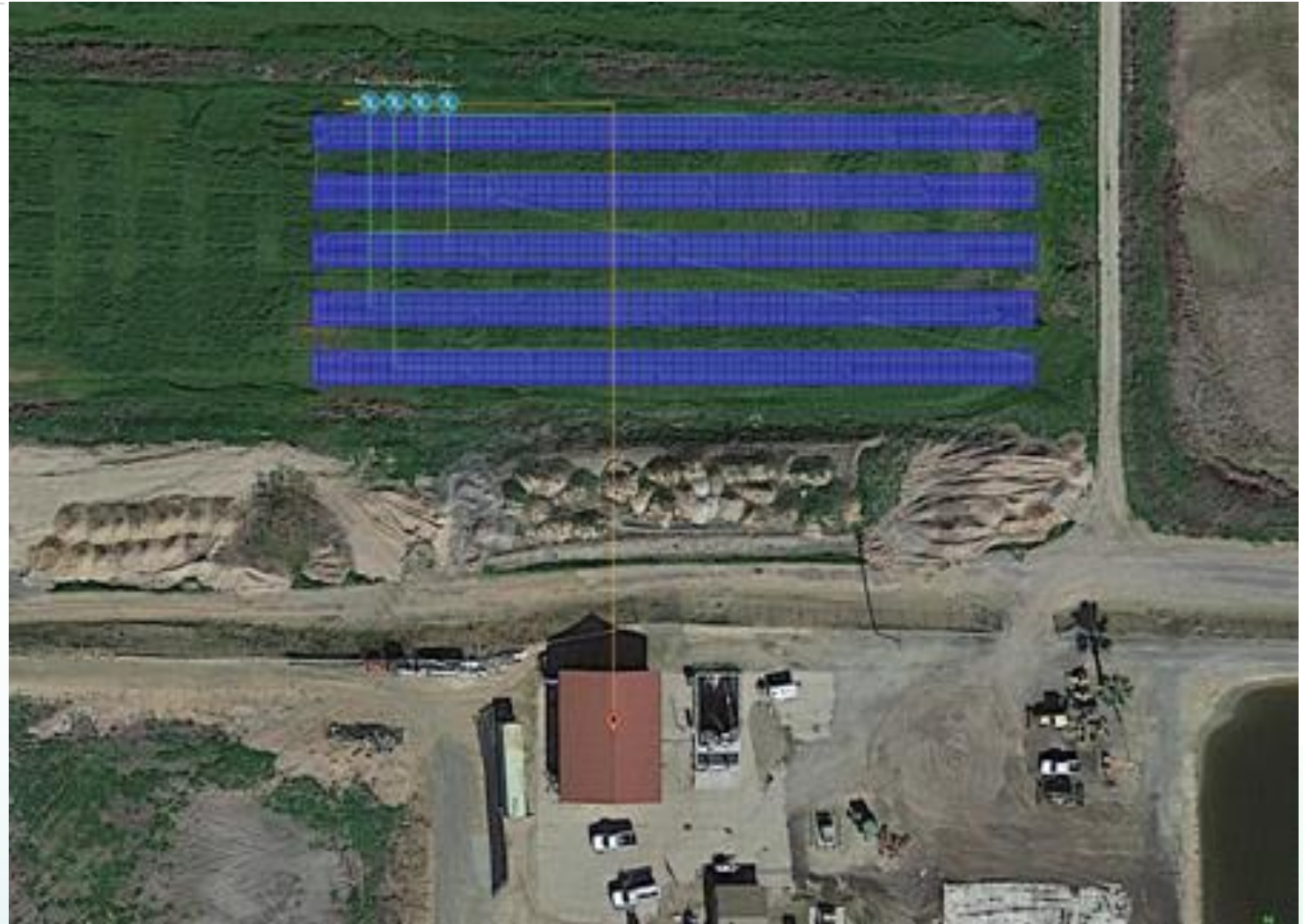
Photo: Wastewater Treatment Plant with Proposed Solar Array
