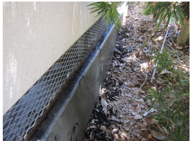
Photograph 36. Transformer oil drainage to soil at eastern equipment pad.
