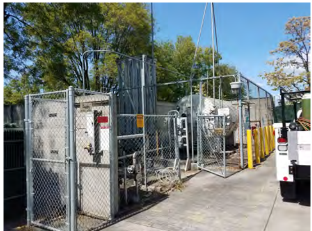
36. Hydrogen gas AST on northwestern property corner.
