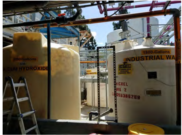
26. Wastewater treatment tanks (Calcium Hydroxide ASTs: 1 2,500-gallon and 3 1,800-gallon_
