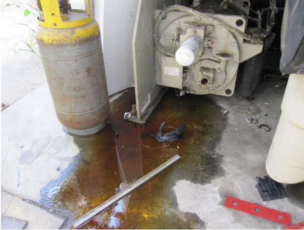
Photograph 25. Oil leak and compressed gas cylinder at chiller on northern equipment pad.
