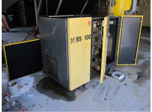
Photograph 26. Oil spillage below vacuum pump.
