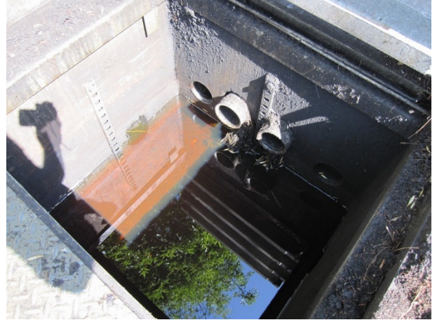
Photograph 32. Apparent transformer oil in electrical vault (within western vehicle drive).
