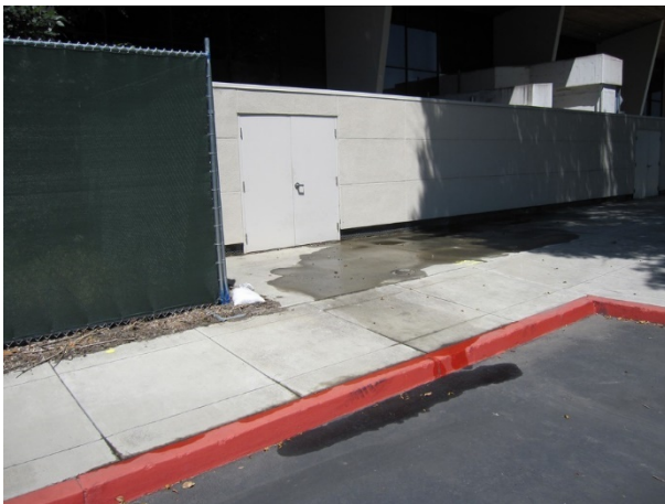
Photograph 35. Transformer oil on pavement from eastern equipment pad.
