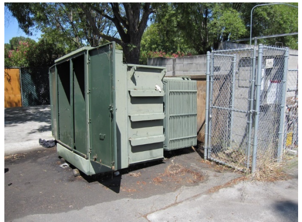
Photograph 34. Damaged transformer and spilled oil on pavement (adjacent to former liquid hydrogen AST)
