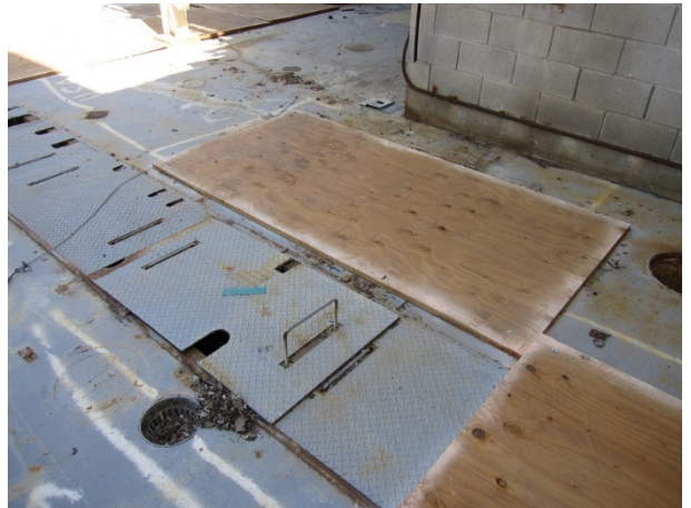
Photograph 16. Acid waste sump and piping trench.
