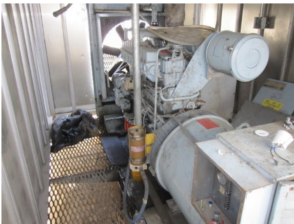
Photograph 23. Emergency generator with diesel AST.
