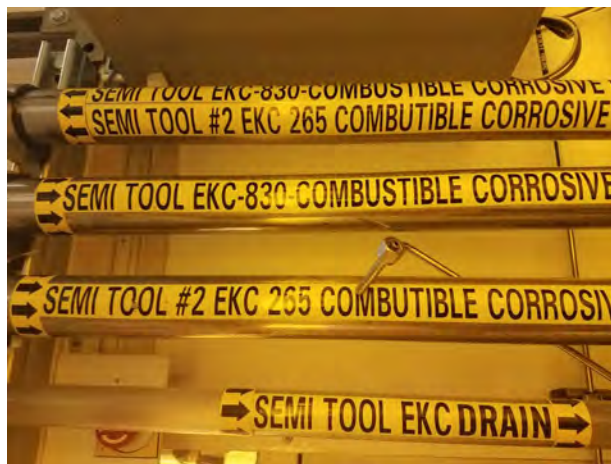
14. Example of drain lines.
