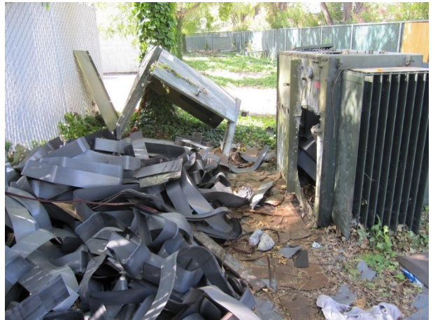
Photograph 28. Damaged transformer (on APN 244-17-005).
