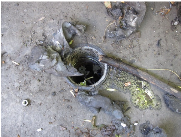
Photograph 33. Apparent transformer oil in electrical conduit.
