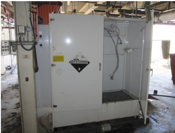
Photograph 21. Corrosives storage cabinet.
