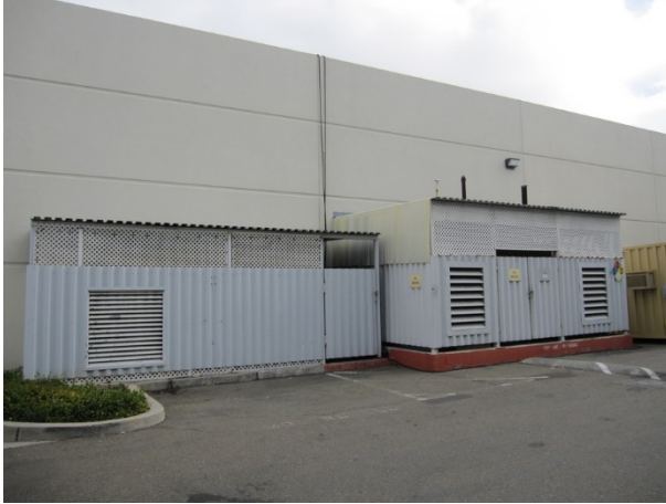
Photograph 7. Emergency generator enclosure.
