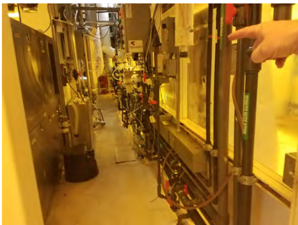
13. Example of a chase (space between lines for accessing plumbing).
