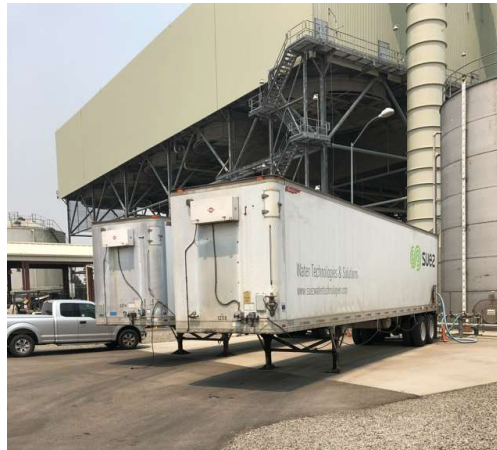
Figure 5: Trailer Mounted Demineralizer Units
