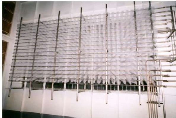
Fog nozzle manifold with multiple feedlines to provide staging
