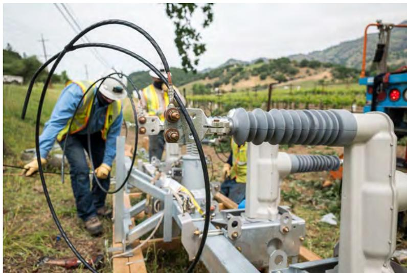
PG&E workers attaching conductors to an automatic circuit recloser in Yountville, Calif., last year.
