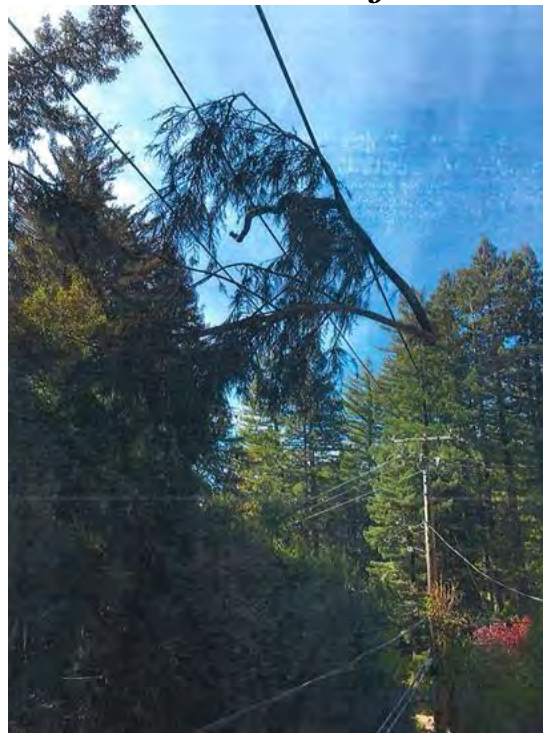
Figure 14 – In Woodside, San Mateo County Branch Flew Onto Primary Conductors
