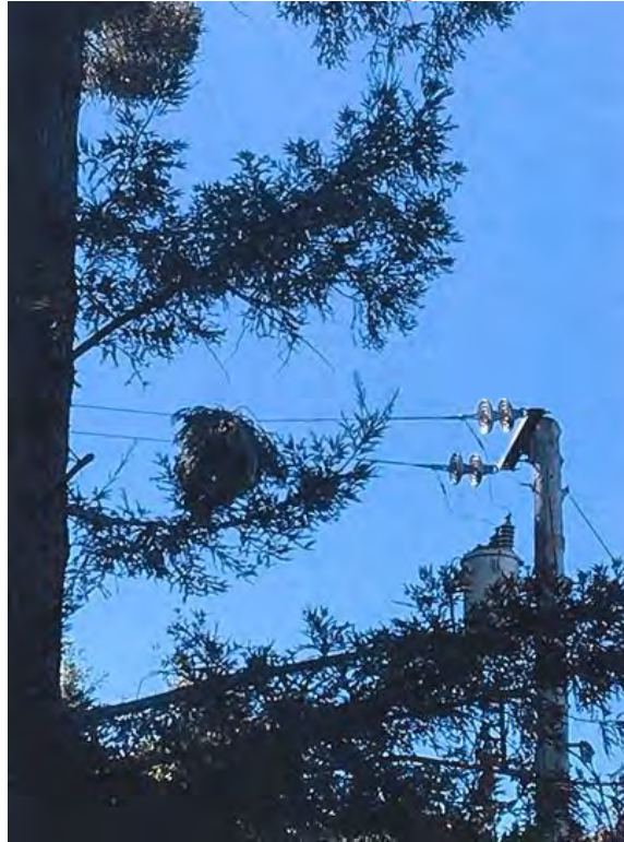
Figure 14 – In Woodside, San Mateo County Branch Flew Onto Primary Conductors
