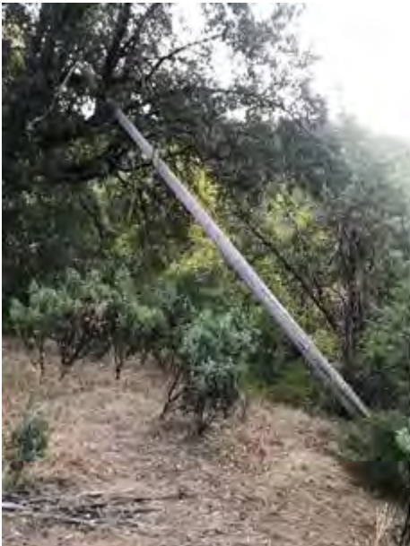
Figure 8 – Near Redding, Shasta County Tree Failed Onto Primary Conductors and Took Down Pole
