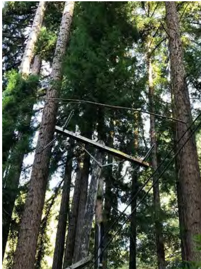
Figure 16 – In Boulder Creek, Santa Cruz County Branch in Contact Cross Phase Conductors
