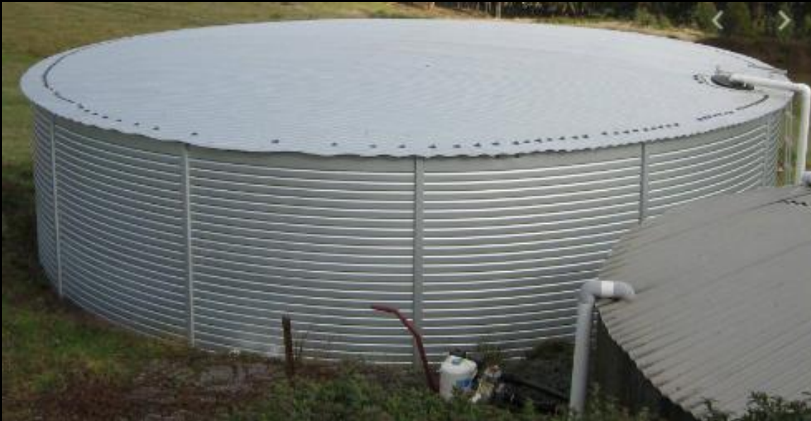
20,000 gallon roof rainwater collection tank
