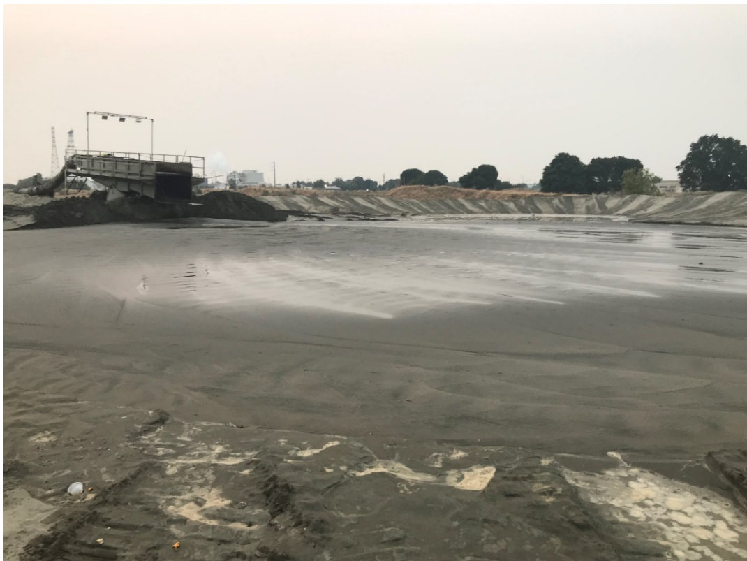
Photo 4. New dredged sand material from the San Joaquin River deposited onto Management Area 2 of the Stamm Unit in October of 2020.
