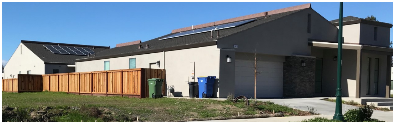
Typical home in Portello subdivision, Windsor, Sonoma County. It features both electric and natural gas services. Photo courtesy R.K. Koslowsky, January 25, 2021
