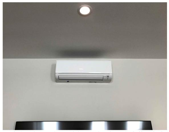
Our ductless split system (a mini-split heat pump), used in our finished lower level, warms the space, eventually. It's visibly mounted high on one wall, is noisier than the gas furnace heating provided upstairs, and blows in your face when sitting on the couch watching television. The companion condenser unit is located outside the house to support the interior electric heating or cooling. During the process, refrigerant [2] is used to optimize the heat exchange.
