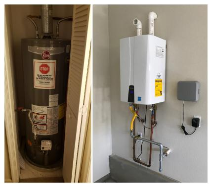
Above left photo: A tank-based water heater, which could be gas or electric. They are easily installed in small garages or very small closets. Above right photo: A tankless natural gas water heater (in white). Very little space in the garage is required to install this reliable ondemand water heating system.
