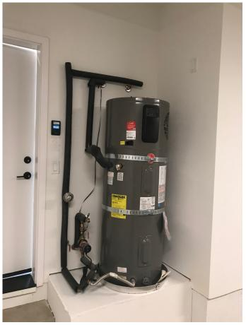
Plan 1's tanked electric water heater element in the garage of a Round Barn townhouse model. The associated shared, heat pump, is mounted on the rooftop to minimize loss of 100-sqaure feet of garage space [3]. Photo courtesy R.K. Koslowsky.
