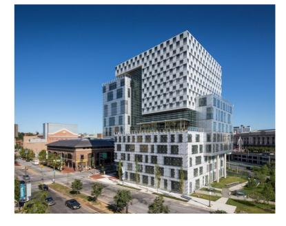
"The facade and atrium design led to passive and active strategies that typically aren't applied in this climate. The building's passive design strategies achieve very high performance and flexibility without the use of PV or solar thermal systems." The windows will be automatically closed when the air condition is on and made available for the users to open and close at will by the manual override switches, when the air condition is off. This saves energy.
