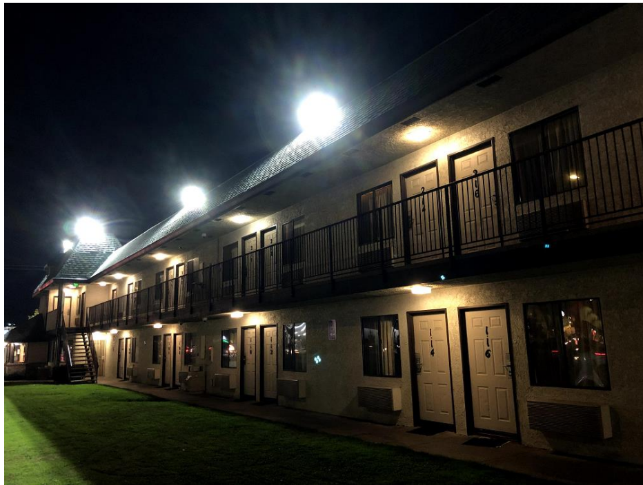
Figure 1 - High color temperature LED floodlights
