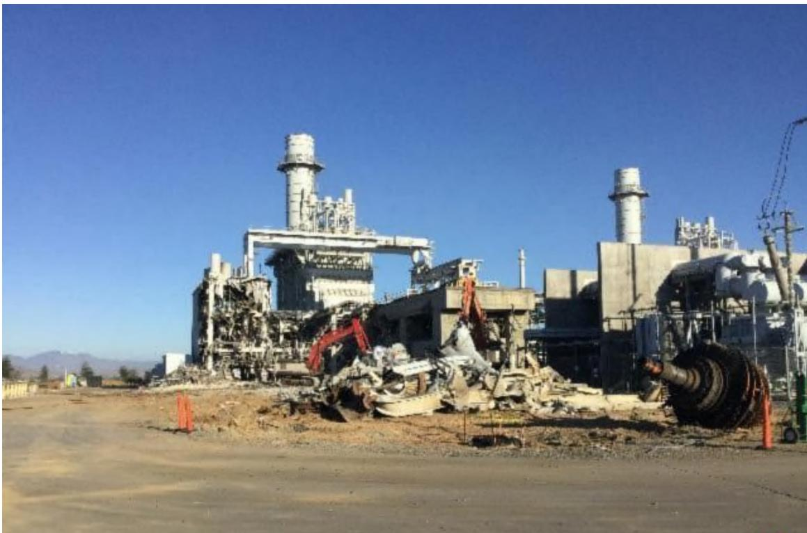
East side of Unit 2, excavators demolishing turbine structures.
