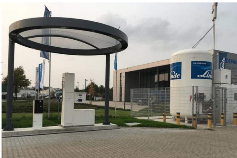
Newly opened hydrogen refueling station in Hannover. Source: Linde.
