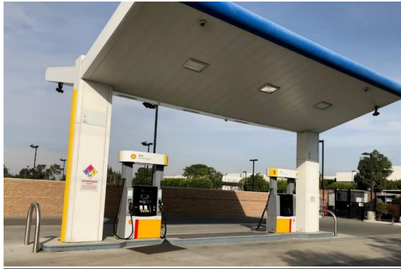
Figure 1 Shell Hydrogen Fueling Station, Torrance, CA (2018)
