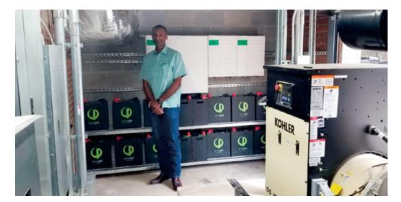
56 kilowatt-hour SimpliPhi battery system at Maycroft Apartments in Washington, DC. Courtesy of SimpliPhi Power
