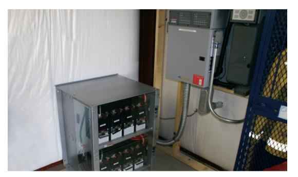
16 kilowatt-hour lead acid battery system at the Cimarron Forestry Office in New Mexico. Courtesy of M. Gaiser, New Mexico State Energy Office
