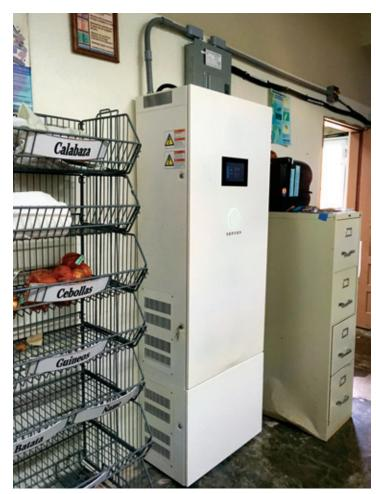
Residential and small commercial battery systems, like this 14-kilowatt-hour sonnen eco 14 battery at a remote school in Orcovis, Puerto Rico, tend to have an average installed cost between \$800 to \$1,000 per kilowatt-hour. Courtesy of sonnen
