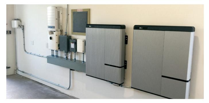
If the battery system is being added to provide backup power during grid outages, another important consideration is verifying that the existing solar inverters can communicate with the new battery-based inverter. Failure to communicate properly could create issues that prevent the
