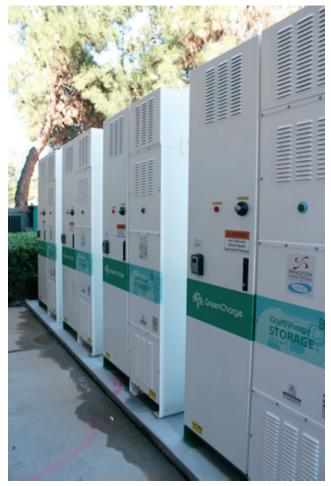
Battery systems in the 100 kilowatt-hour to 500 kilowatthour range, such as this system at a Safeway supermarket in San Jose, CA, typically cost less than smaller systems, around the \$600 to \$800 per kilowatt-hour range. Courtesy of ENGIE
