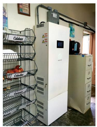
Residential and small commercial battery systems, like this 14-kilowatt-hour sonnen eco 14 battery at a remote school in Orcovis, Puerto Rico, tend to have an average installed cost between \$800 to \$1,000 per kilowatt-hour.
