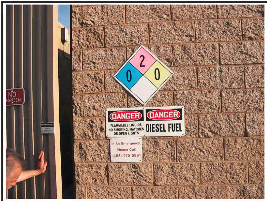
Photograph 11: Appropriate hazard placarding is present outside the emergency generator enclosure on the south side of Building 700.
