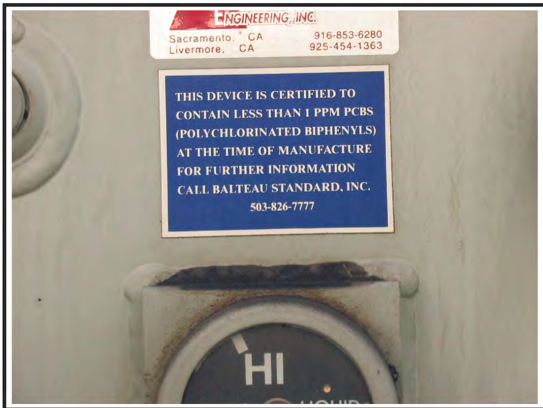
Photograph 9: The transformer units are identified as “Non PCB” units.
