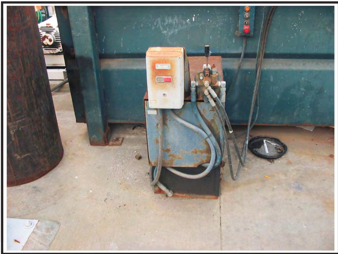
Photograph 7: Looking at the hydraulic trash compactor equipment located outside Building 750. No leaks or stains were present.
