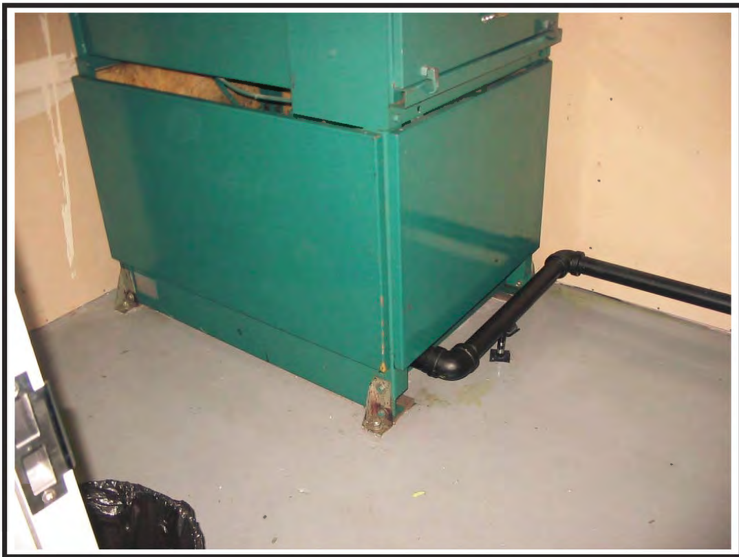
Photograph 13: There were no leaks or stains observed around the hydraulic elevator equipment in Building 750.
