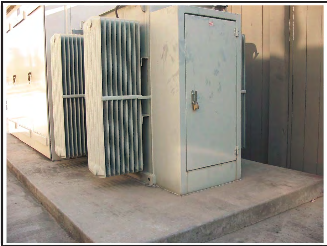
Photograph 8: Looking at one of the pad-mounted electric transformers. No leaks or staining were observed around any of the on-site transformers.
