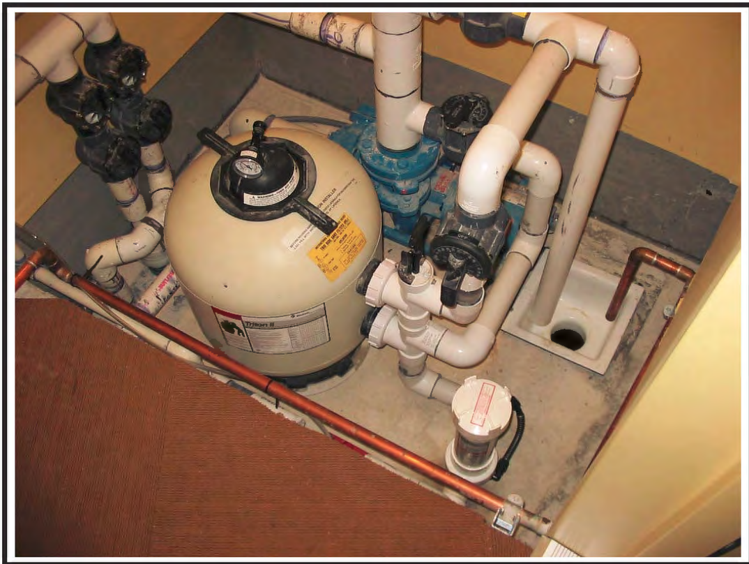
Photograph 14: Looking at one of two water feature circulating equipment in Building 700. Three inch chlorine tablets are used to sanitize the water.
