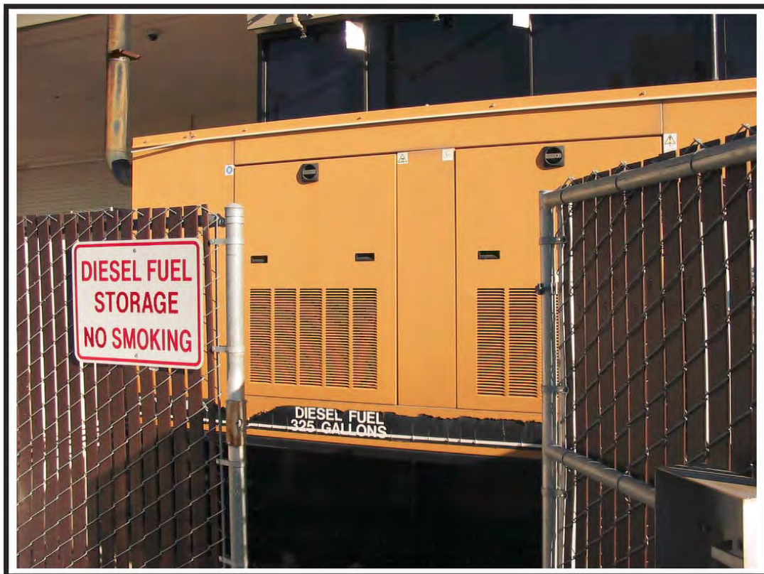
Photograph 10: Looking at the diesel powered emergency generator installed outside Building 750. No issues were identified with the fuel storage.
