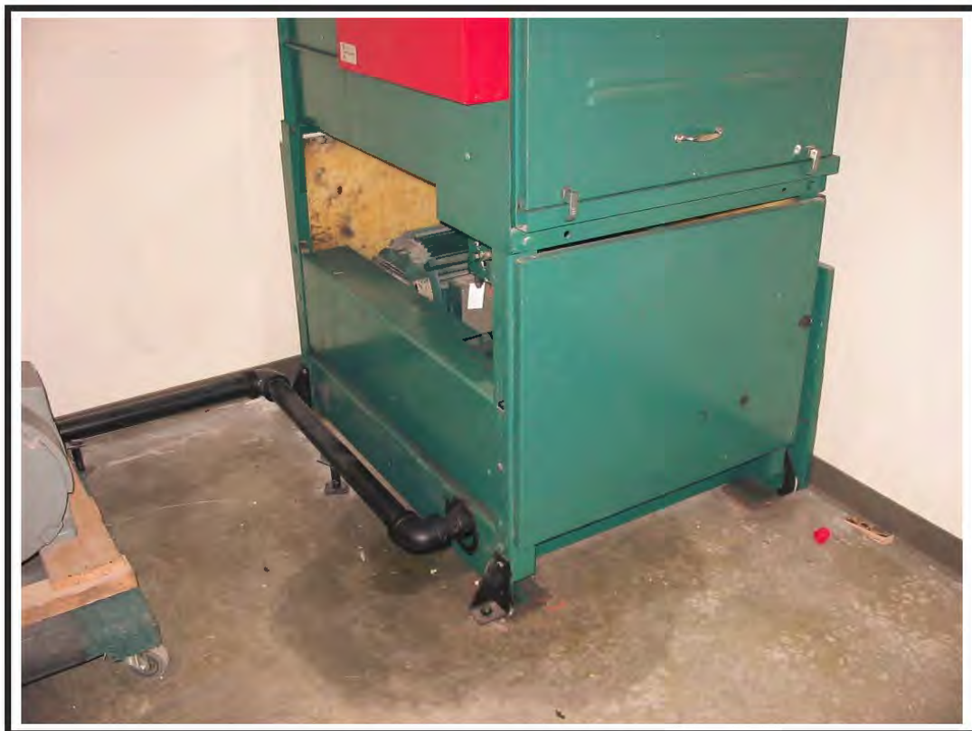
Photograph 12: Minor staining ( de minimis condition) was observed on the concrete flooring at the hydraulic elevator equipment in Building 700.
