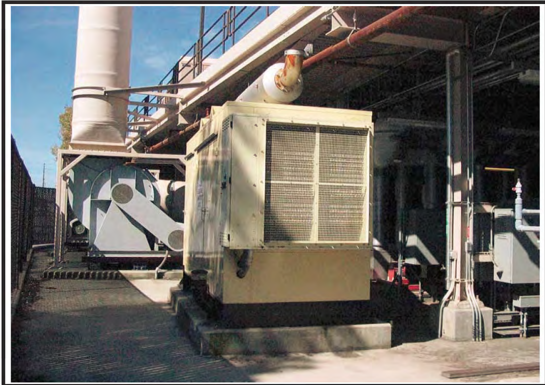
Photograph 18: Looking at the new diesel-powered emergency power generator located on the south side of Building 800. Since the motor is still wrapped in plastic, the generator has never been used.
