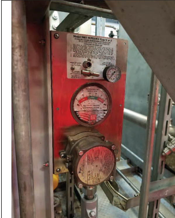
Photo 3 Purge system components
