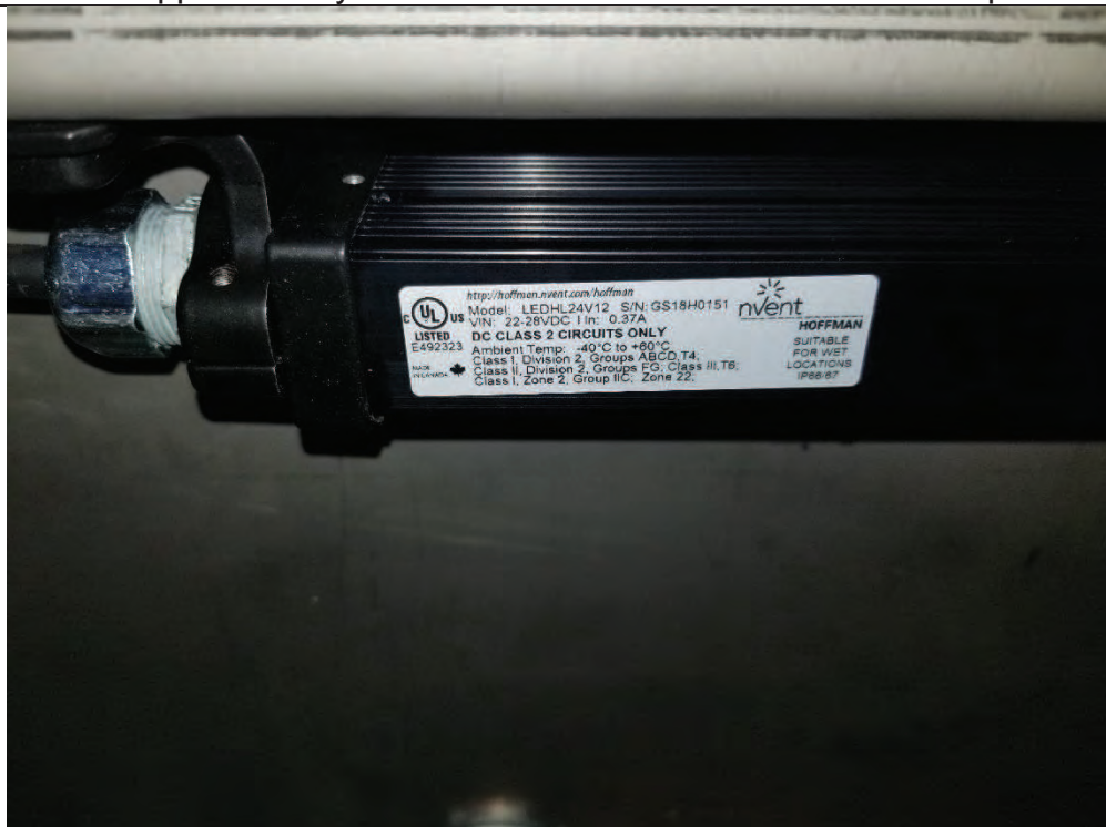
Photo 6 Panel light-marked for use on class 2 circuit only.
