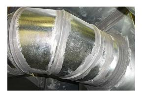
Figure 21: Duct with mastic applied.
