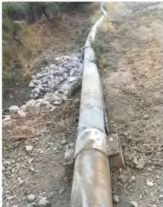
Injection Line Straightening and Culvert Repair
