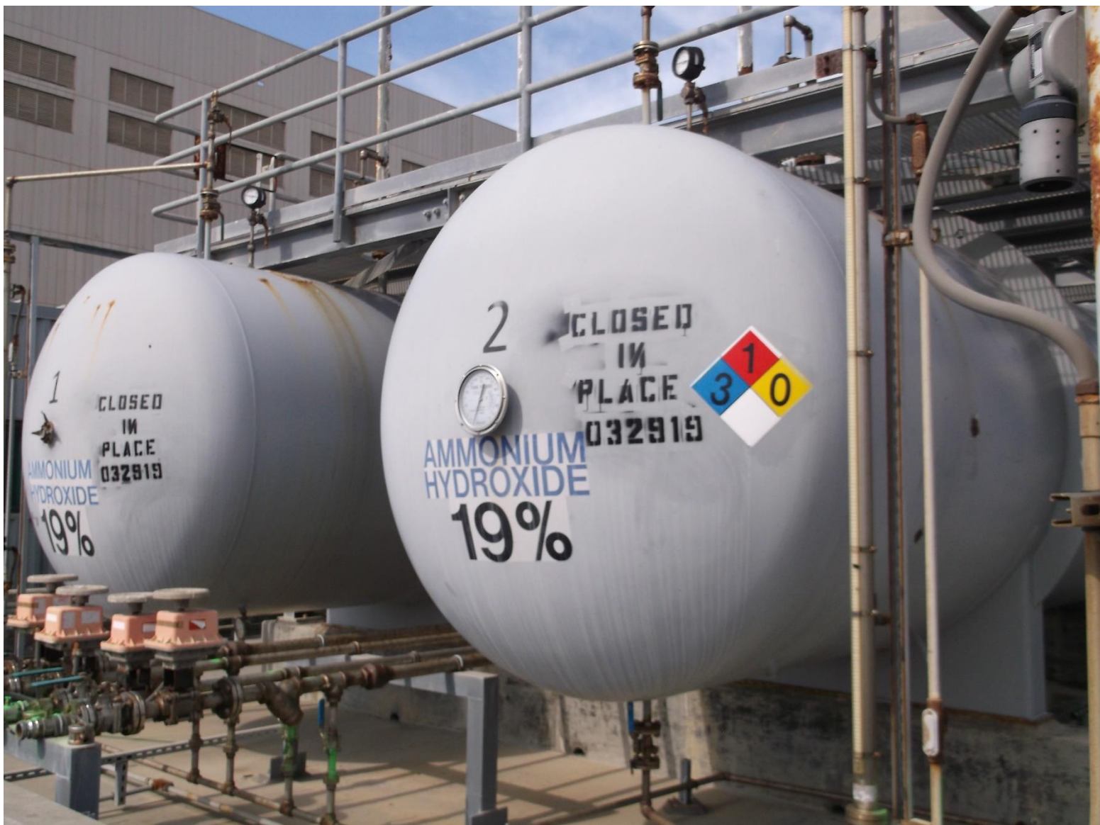
Photo #4: Ammonia Storage Area disconnected and verified tanks purged (cleaned) prior to cut and haul away
