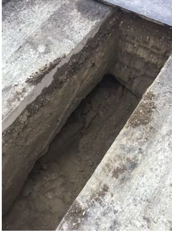
East. Sinkhole feature discovered when moved into the intersection at Ball Ave (3 ft depth)
