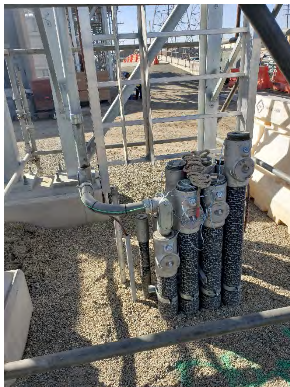
UG to OH Raceway Transition
