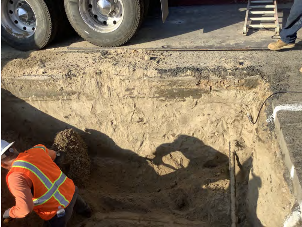
Natural gas linear at 30" main tie-in with upper 4 feet backfill stratigraphy in view featuring numerous clouds of oil-impregnated sand. View toward north from 0408860mE and 3745607mN
