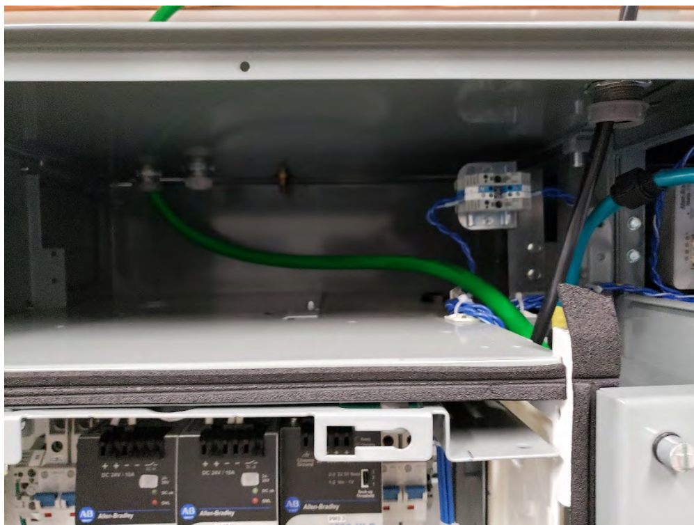
MCC Ethernet Connection
