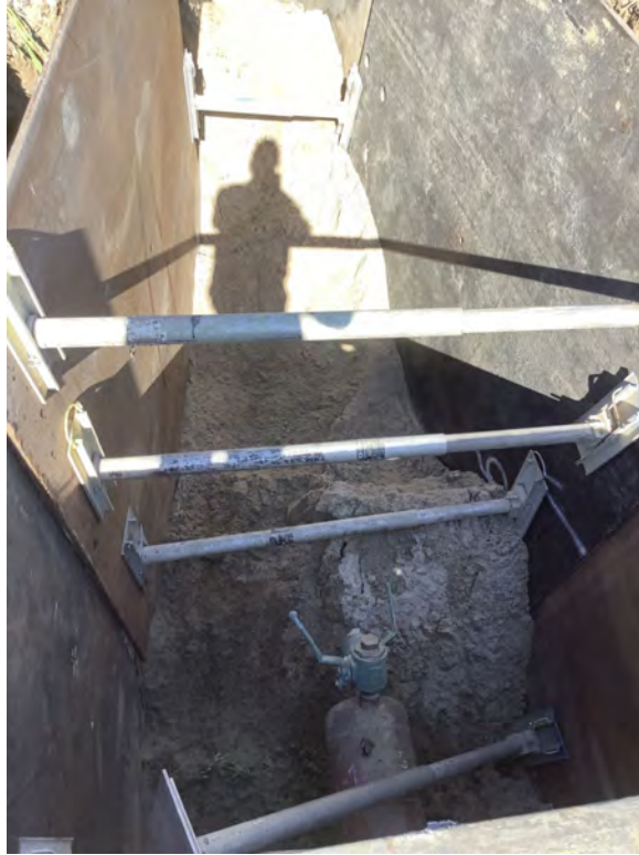
17: PWR 08-11-19-01 sub grade lithology/sample location station 00+18' and 8 1/2 feet deep in light gray-tan moist fine to coarse sand with trace of gravel.
