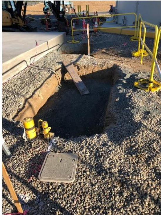
Photo 16: Excavation with escape ramp placed inside on October 12, 2018.
