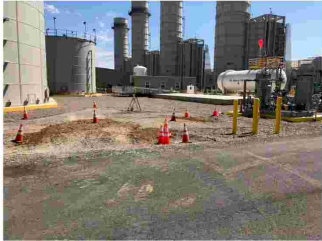
Photos 7 and 8. Photographs showing removal of aggregate base and backfilled potholes in the Project area.
