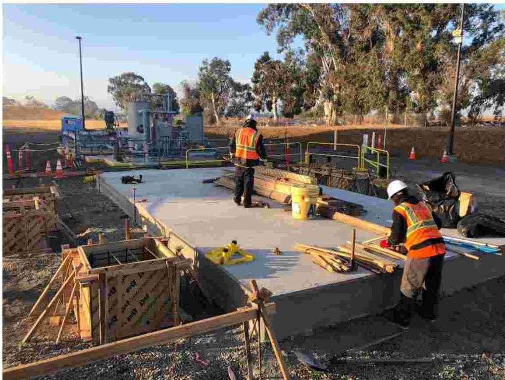
Photo 11: Forms and rebar being constructed for concrete pipe supports on October 25, 2018.
