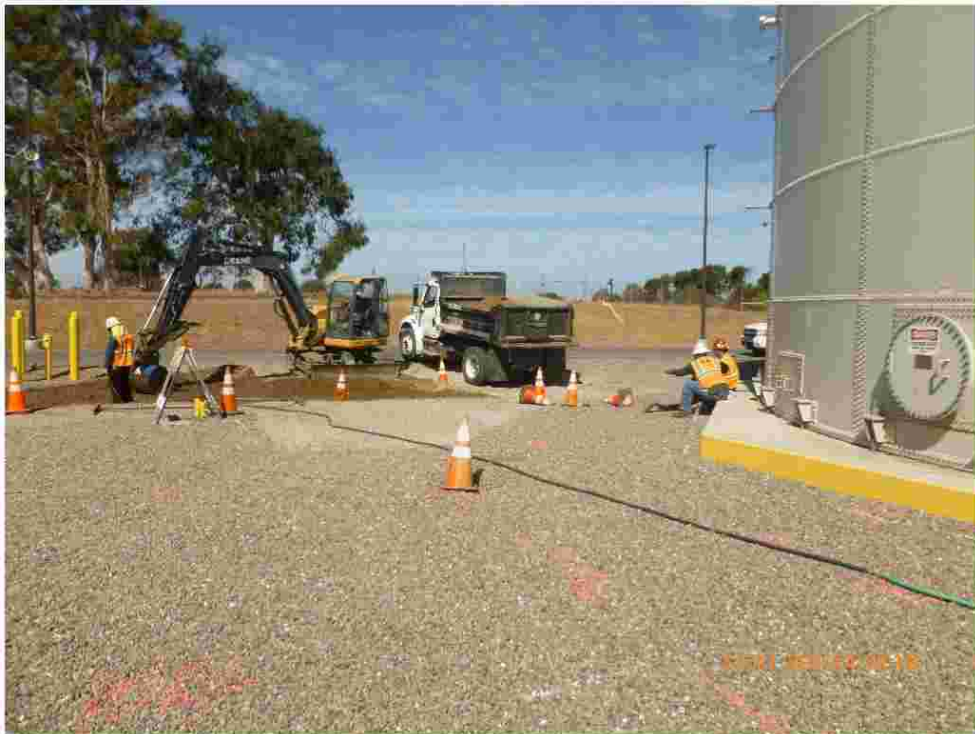
Photo 4: Excavation of relief trenches and foundation pad for the fire pump on September 14, 2018.
