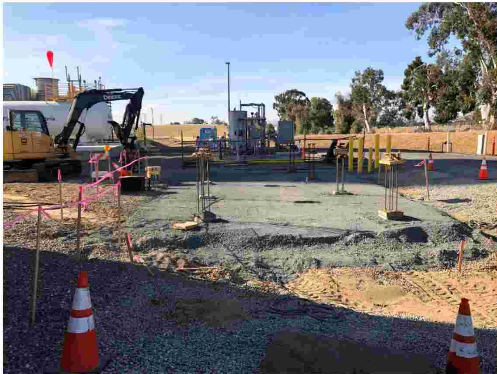
Photo 9: Foundation pad for fire pump station on September 27, 2018.
