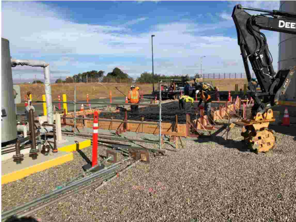
Photo 10: Forms and rebar being constructed for the fire pump foundation pad on October 4, 2018.
