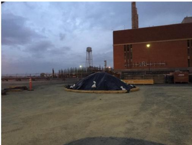
Photos 21 through 23: Stockpiles are all covered ahead of storms on November 21, 2018.
