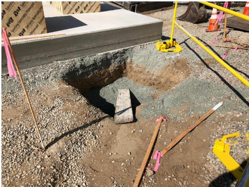
Photo 17: Excavation with escape ramp for wildlife, October 18, 2018.
