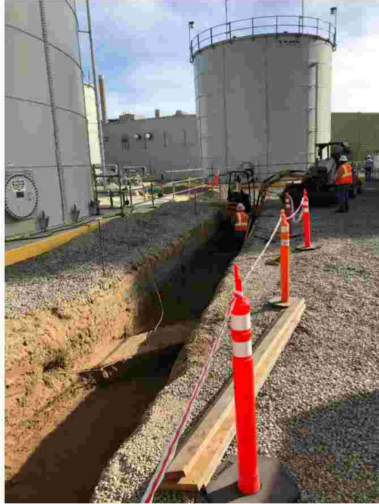
Photo 12: Excavation for pipeline on November 1, 2018.
