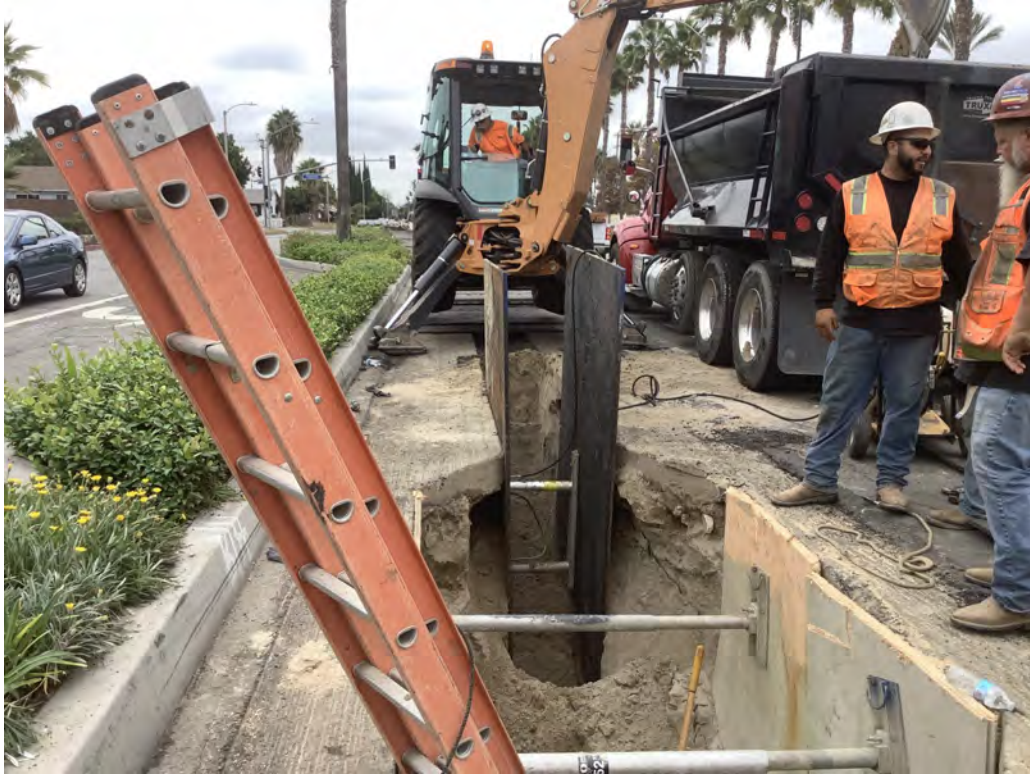
South, start of machine excavation at 2+75. Depth going to max 9 ft. Soft sand starts at 2 ft and continues all the way down.
