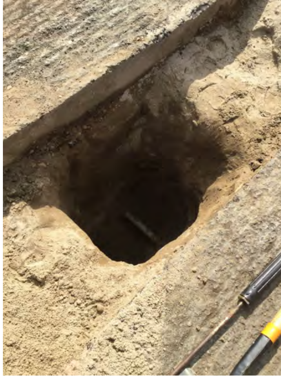
Pothole at Buena Park Downtown; existing pipeline is at approximately 4ft down. 3 feet of fill underlaid by clean medium sands of Holocene age.
