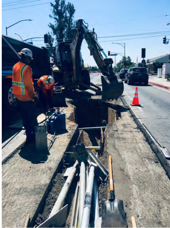
Trenched length for the day. Cave-in observed during trenching activity near Station # 2640
