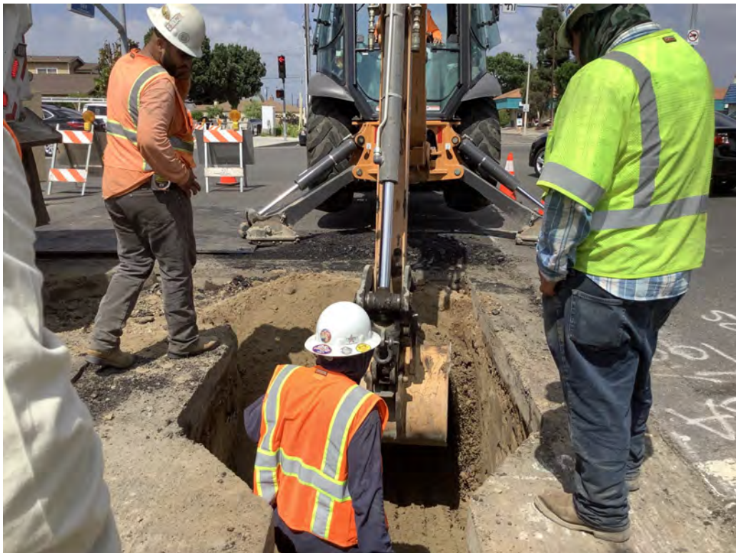
North, crew excavating around water main at intersection. (1+45)
