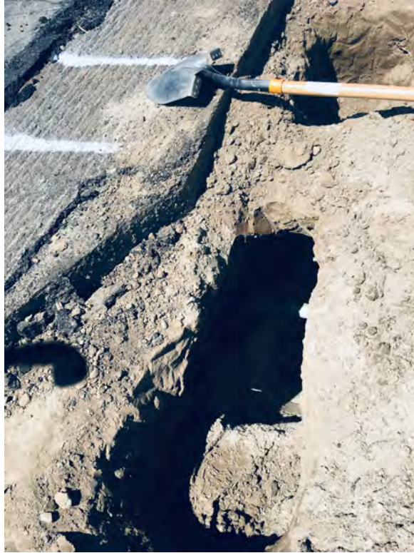
Hand dug holes for utilities down to about 2-3 ft.
