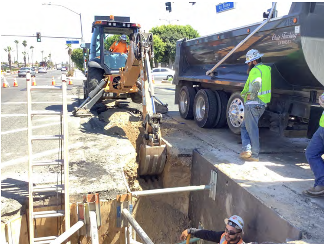
East, southeast crew continuing at 0+75 digging down to 8 ft depth.
