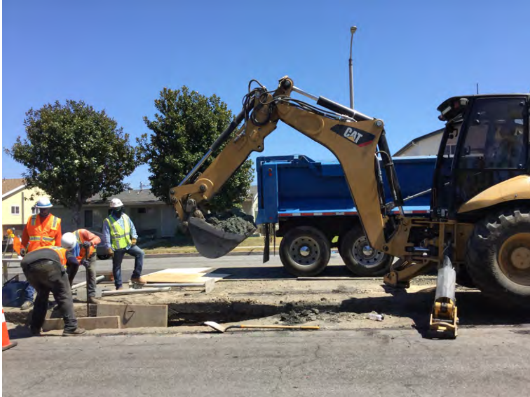
Trenching for gas pipeline installation in HS 21.
