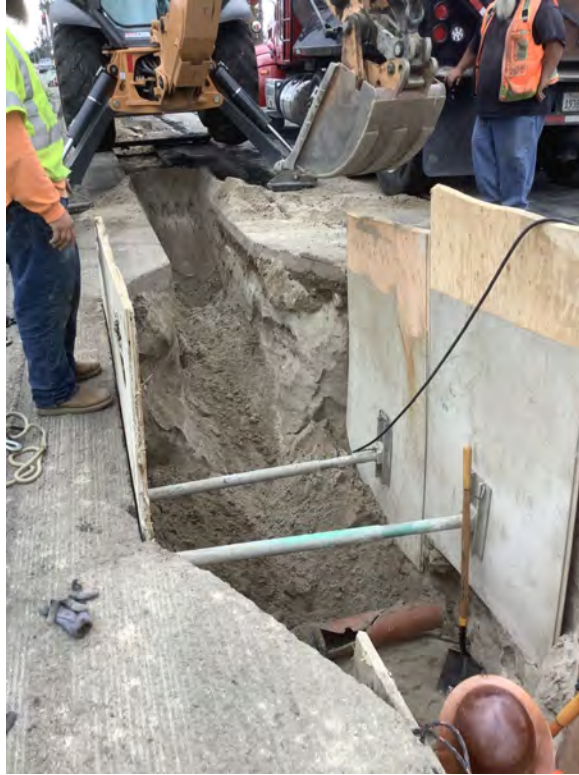
South, crew hit an unmarked sewer pipe and are in the process of excavating around it to determine next step.
