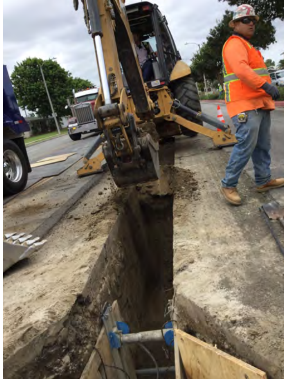
Trenching for gas pipeline installation between HS 22 + 00 and HS 22 + 50.
