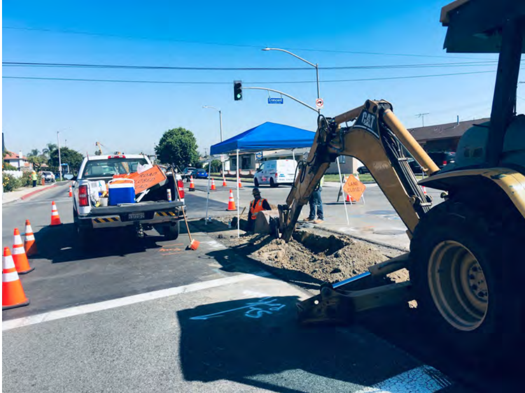
Pot holing for multiple underground utilities at the intersection of Crescent Ave and Dale Ave near Station # 2750
