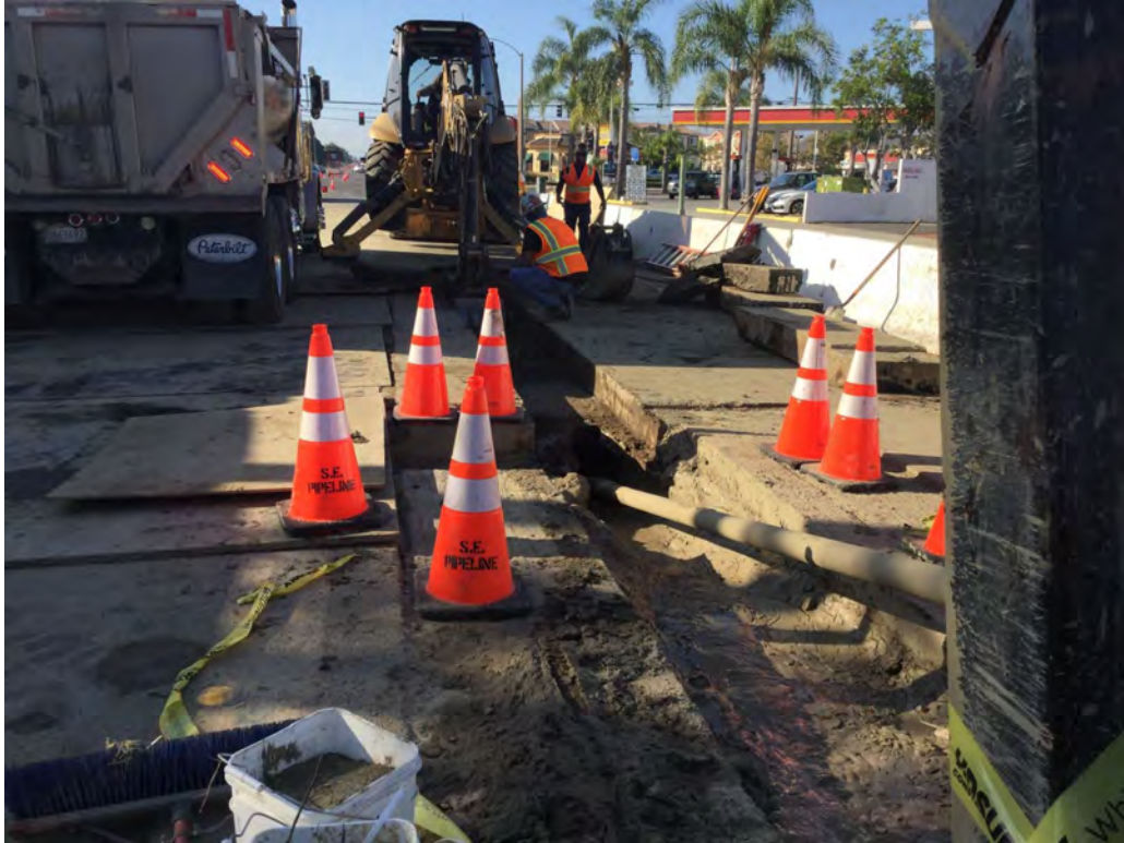
South, HDD backhoe being used to help excavate around HDD drill shaft. @ Lincoln and Dale Ave.
