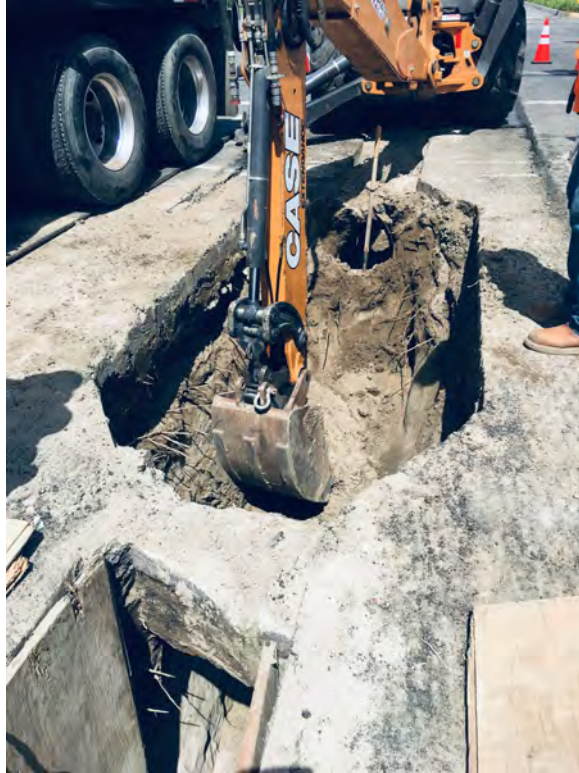
Trenching for Bell-hole north of Station # 680
