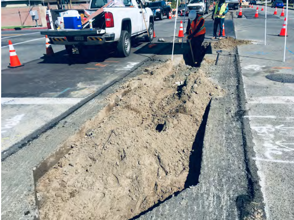
Pot holing for multiple utilities just south of Station # 2750 intersection of Crescent Ave and Dale Ave.
