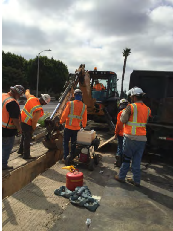
Excavations at La Palma and Dale; very sandy at depths of 7-8ft within Holocene alluvium
