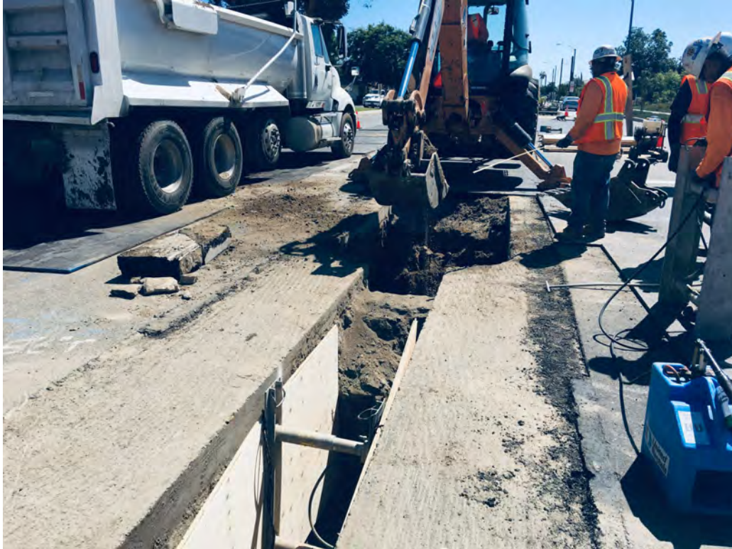
Trenched section from near Station # 2750 with maximum depth of about 13 ft.
