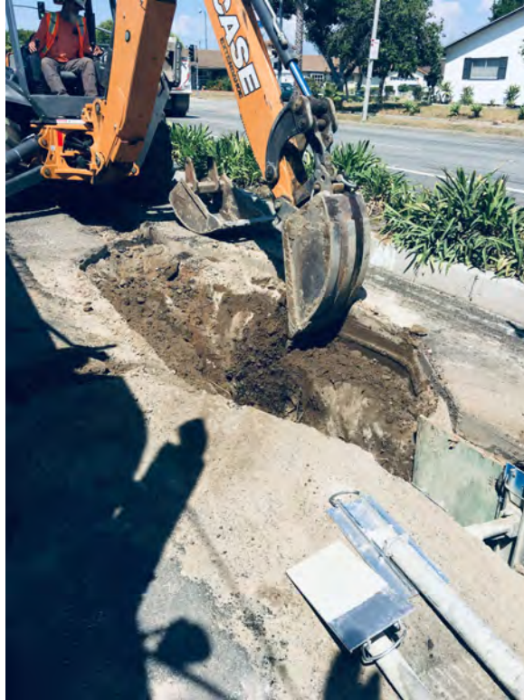
Trenching of Bell-hole north of Station # 825
