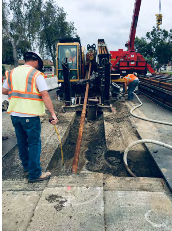
HDD operation in progress with Entry Pit close to Station # 5125
