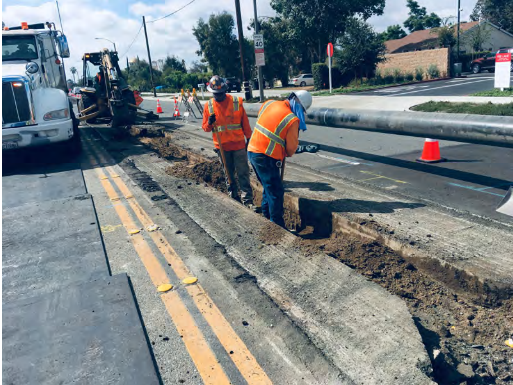
Pot holing for utilities near Station # 3050
