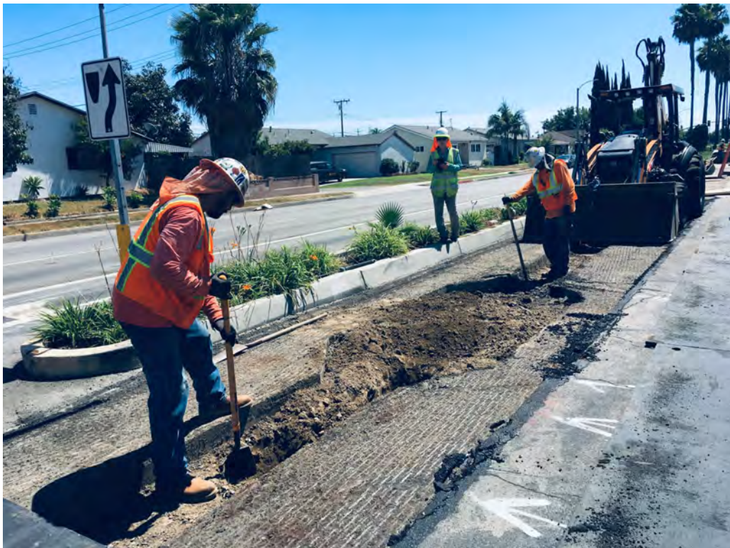
Hand digging to locate underground utilities just north of Station #700
