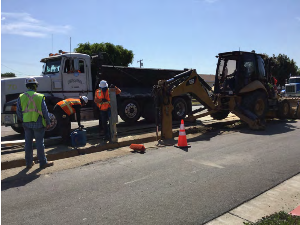
Trenching south on Dale Ave between Stations 18 and 19 for gas pipeline installation.
