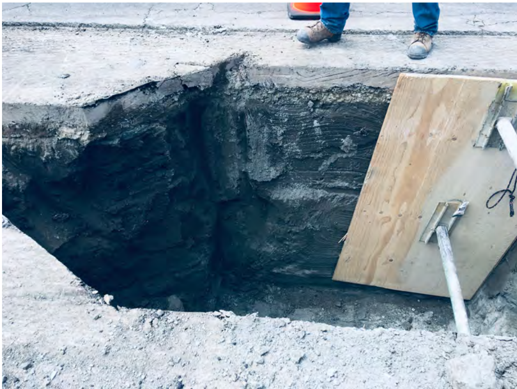
Greenish gray friable silty sands probably of marine origin just south of Station # 2400
