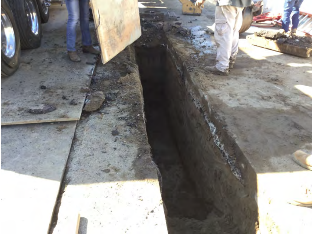
South, HDD dug down to drill, 6 ft.
