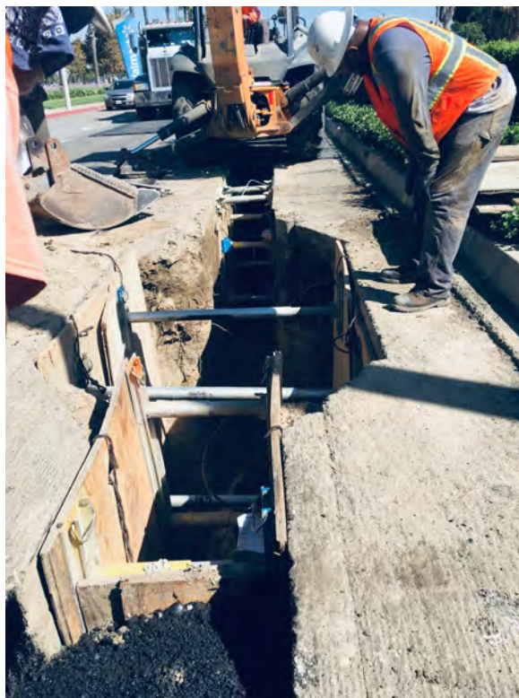
Trenching of Bell Hole north of Station # 900
