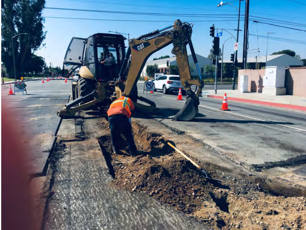
Pot holing for underground utilities near Station # 2640
