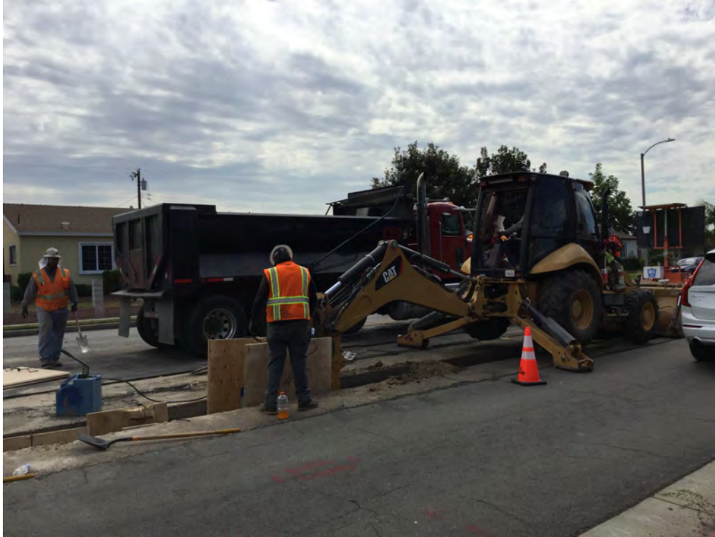
Trenching for gas pipeline in HS 19 headed towards 20.
