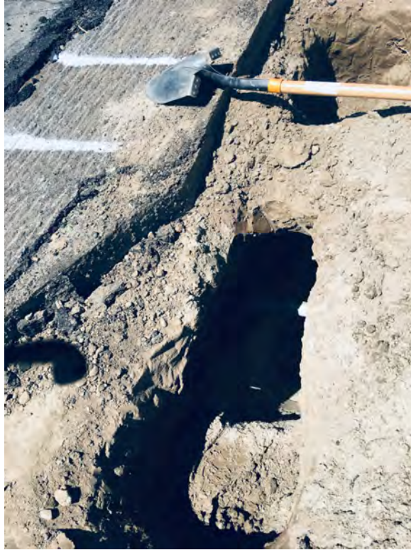
Hand dug holes to locate underground utilities down to about 2-3 ft just north of Station # 700
