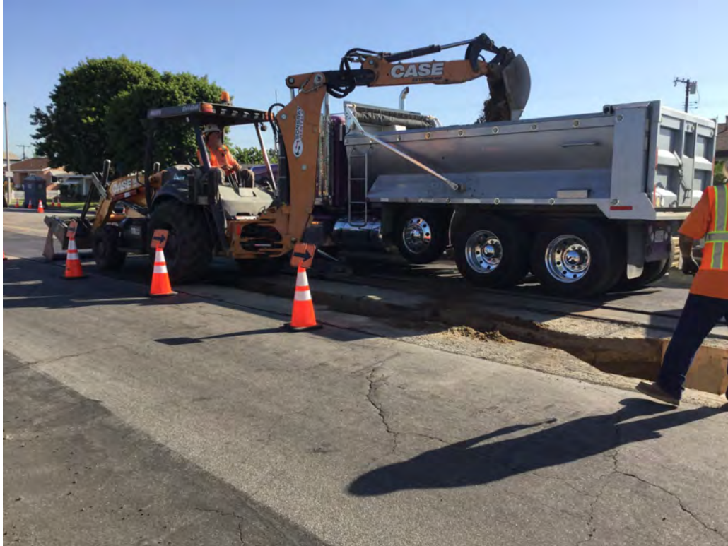
Excavation starting with 5 ft wide section between 25+80 and 25+85 that they could not finish yesterday. (7 ft depth). East
