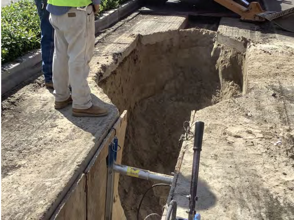
South. Crew excavating down to 7 ft at bel hole (3+20)
