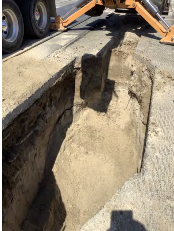
North, inside of trench at tamarack and Dale. Sand is starting to become soft
