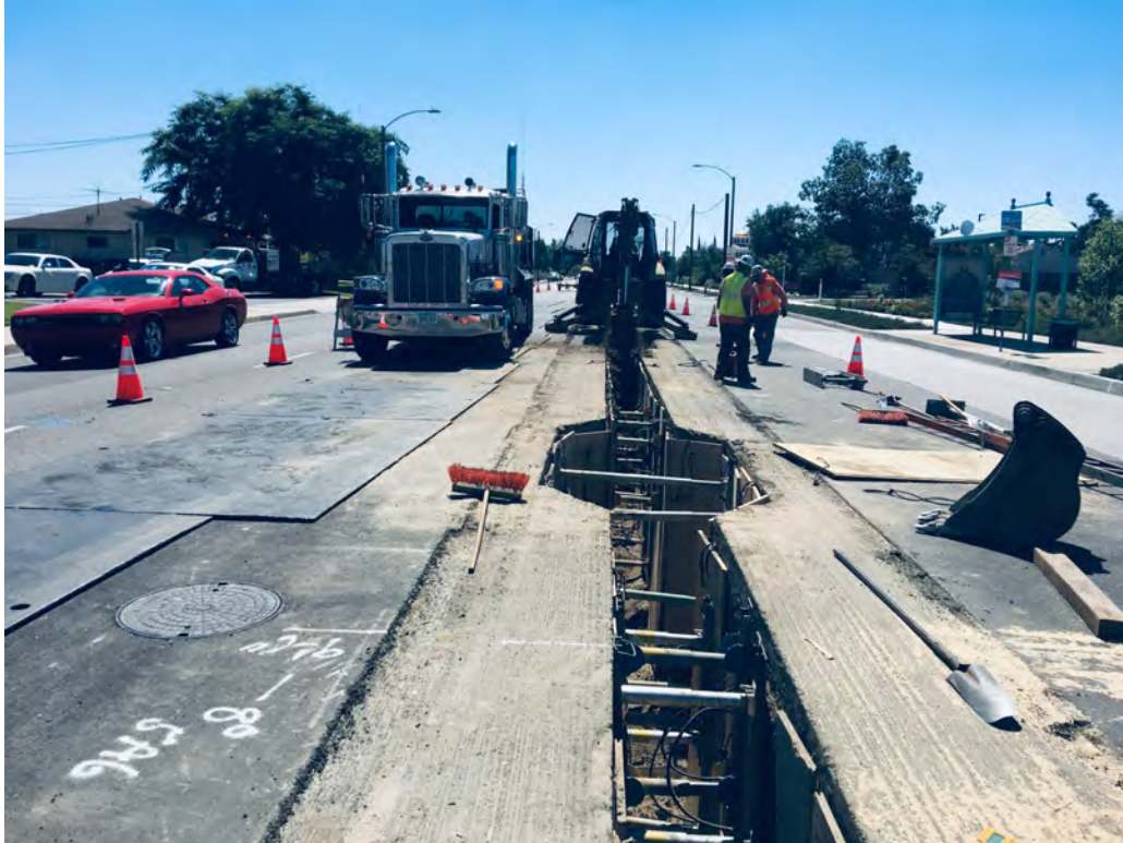
Trenched section south of Station # 2900 down to max depth of about 10 ft.
