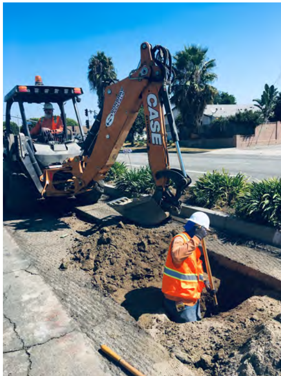
Pot holing for electrical conduit down to max depth of 5 ft north of Station # 900
