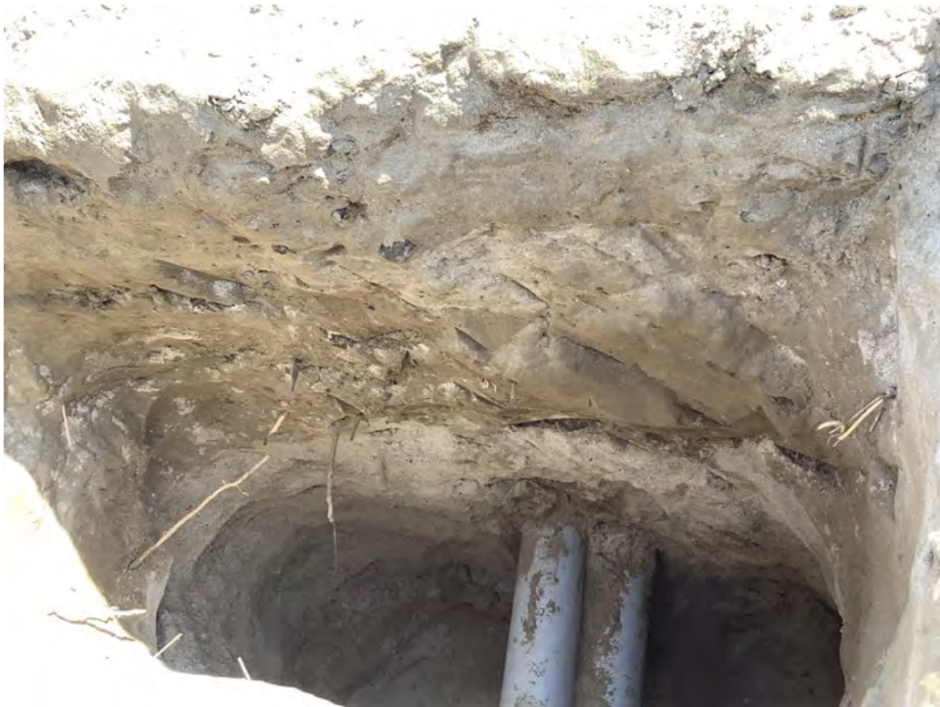
East. Pothole to 57 inches with pipes 12 inches above bottom. All fill.
