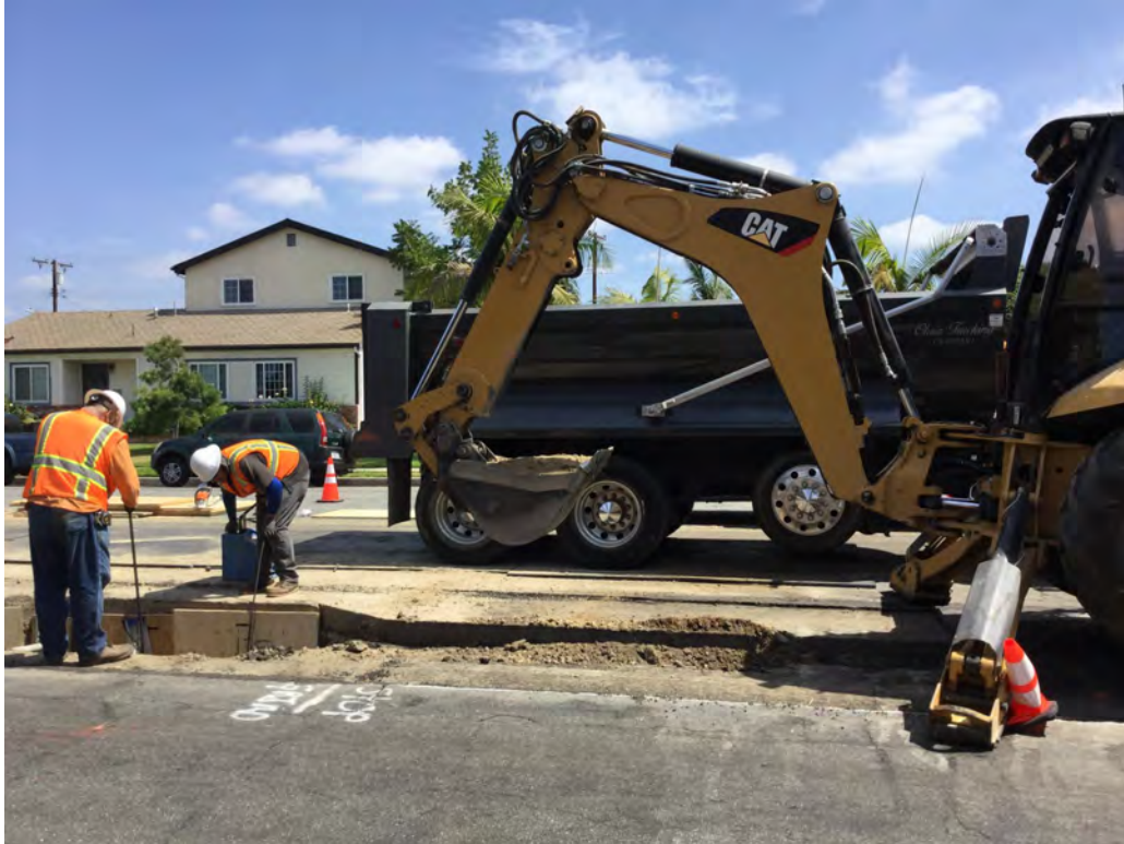
Trenching for gas pipeline installation in HS 22 + 00.
