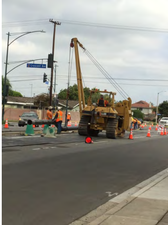
Crew laying pipe just NW of Crescent Ave and Dale intersection.
