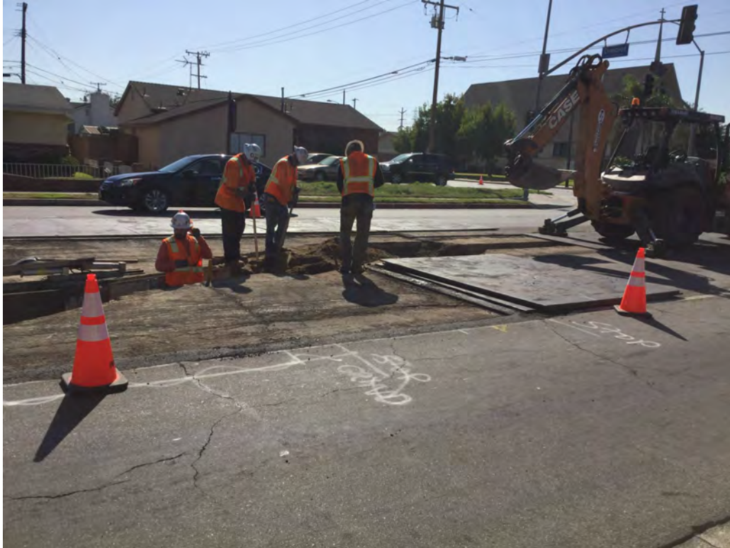
Potholing at 26+50 for gas utilities. East
