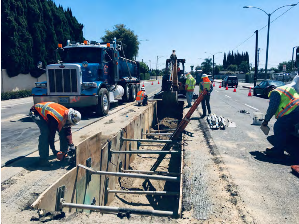
Trenching for HDD EXIT POINT just south of Station # 6350
