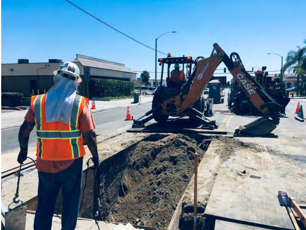
Trenching for HDD mud pit at south end.
