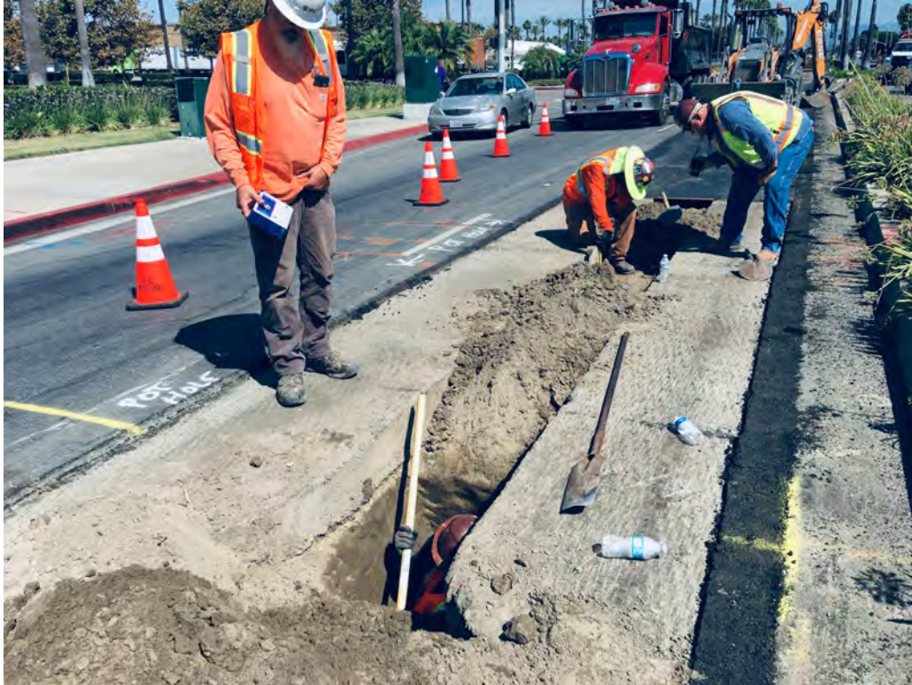
Potholing south end of today's trenching down to maximum depth of 6ft. Dug in all predisturbed sediments 70% and 30% unconsolidated sands.
