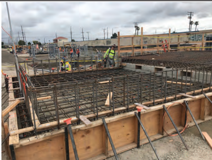
Wire Fabric for weep holes @ Bridge Wingwalls
