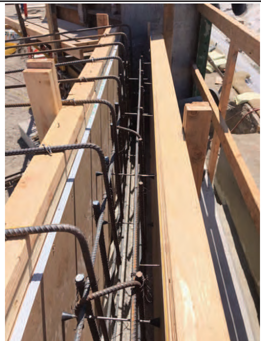
e/Abut top section wall reinforcement inspection
