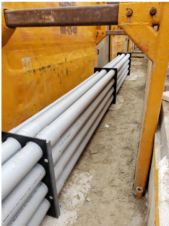
5/14/2019: 66-kV Duct Bank
