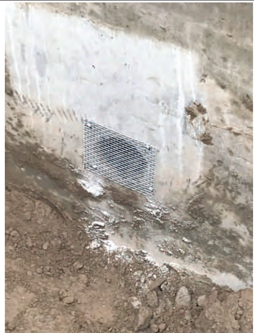
Wire Fabric installed at Wingwalls
