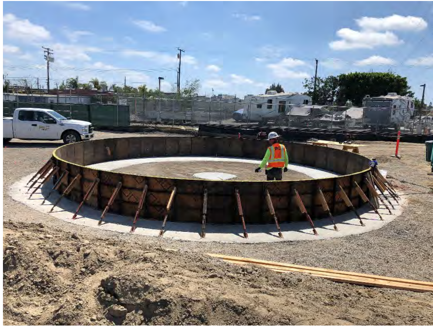
3/26/2019: Demin Tank Formwork
