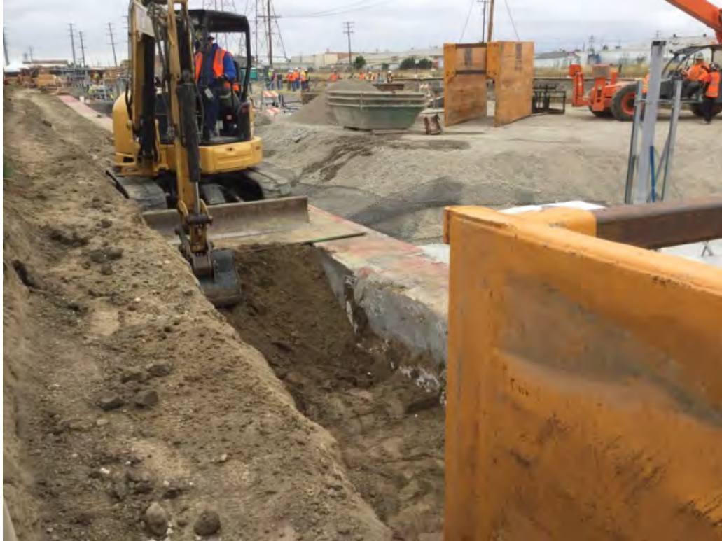
Mini ex excavating along south end of parcel 1
