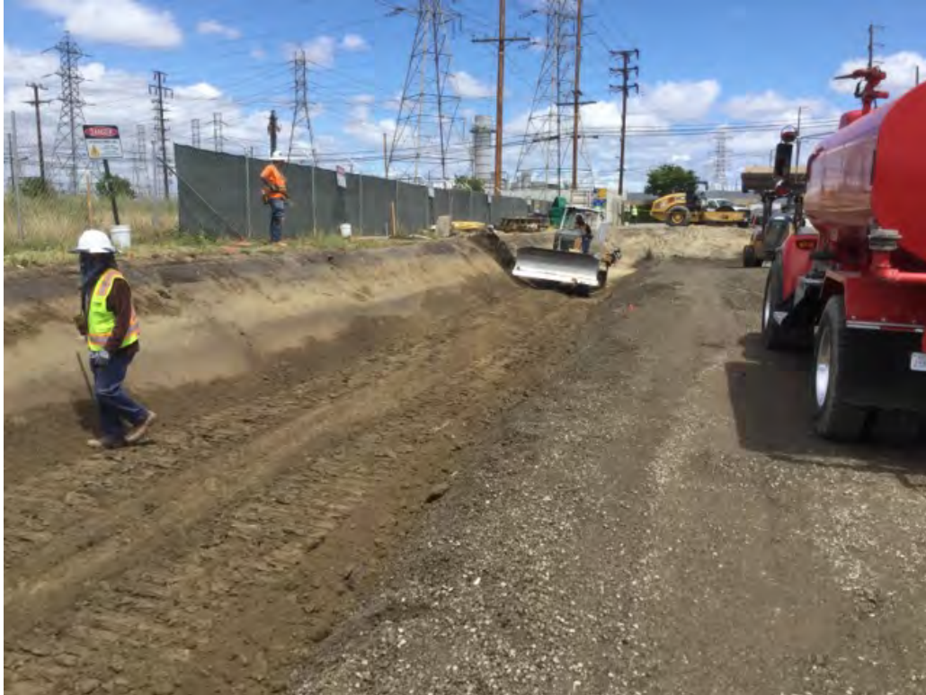
Dozer cutting the north wall for a Duct bank
