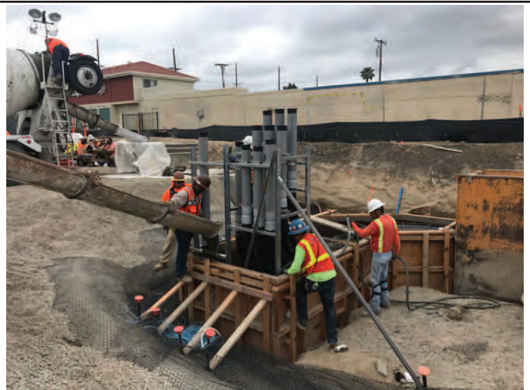
Wire Fabric installed at Wingwalls
