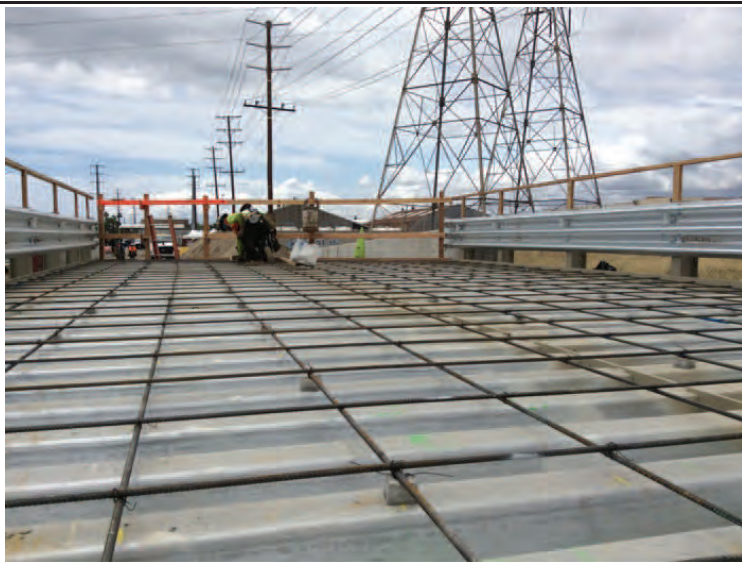
GSU Foundation reinforcement installation
