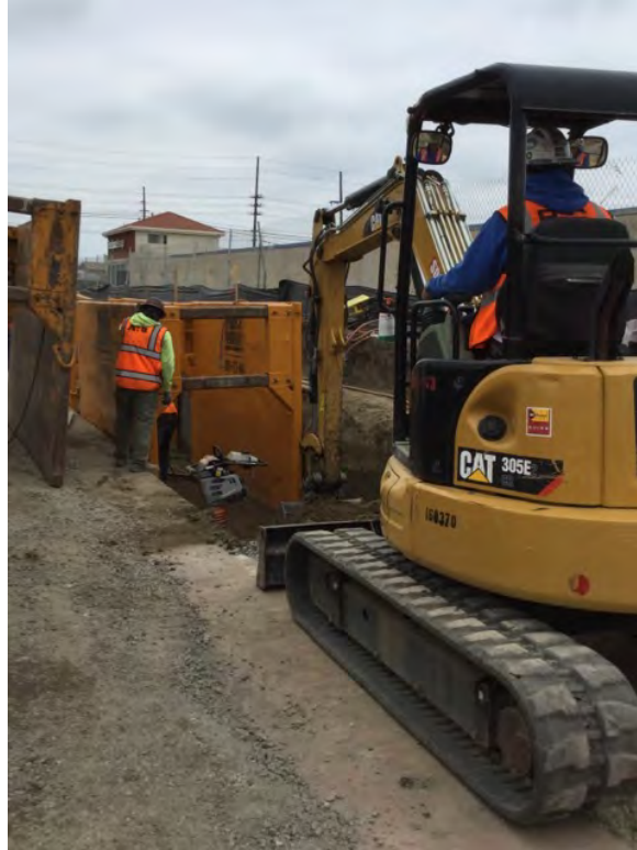
Miniex excavating along south end
