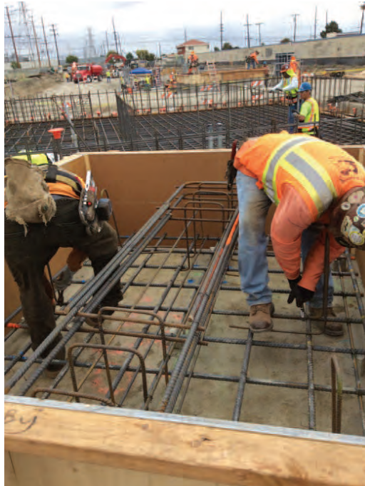
Reinforcement installed @ Utility Rack #2
