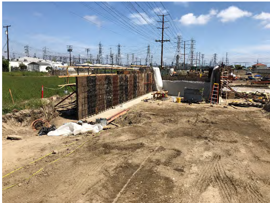
3/26/2019: Bridge Formwork and Reinforcement
