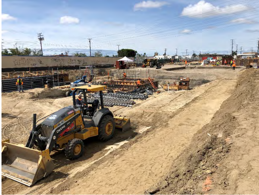
3/27/2019: NH3 Formwork and Rebar, Duct Bank Along South, and Substation Earthwork
