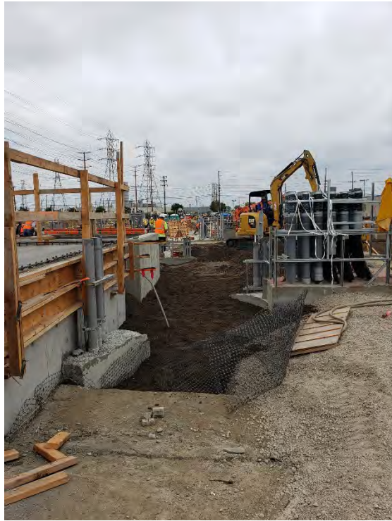
5/14/2019: NH3 Area Conduit Stub-Ups
